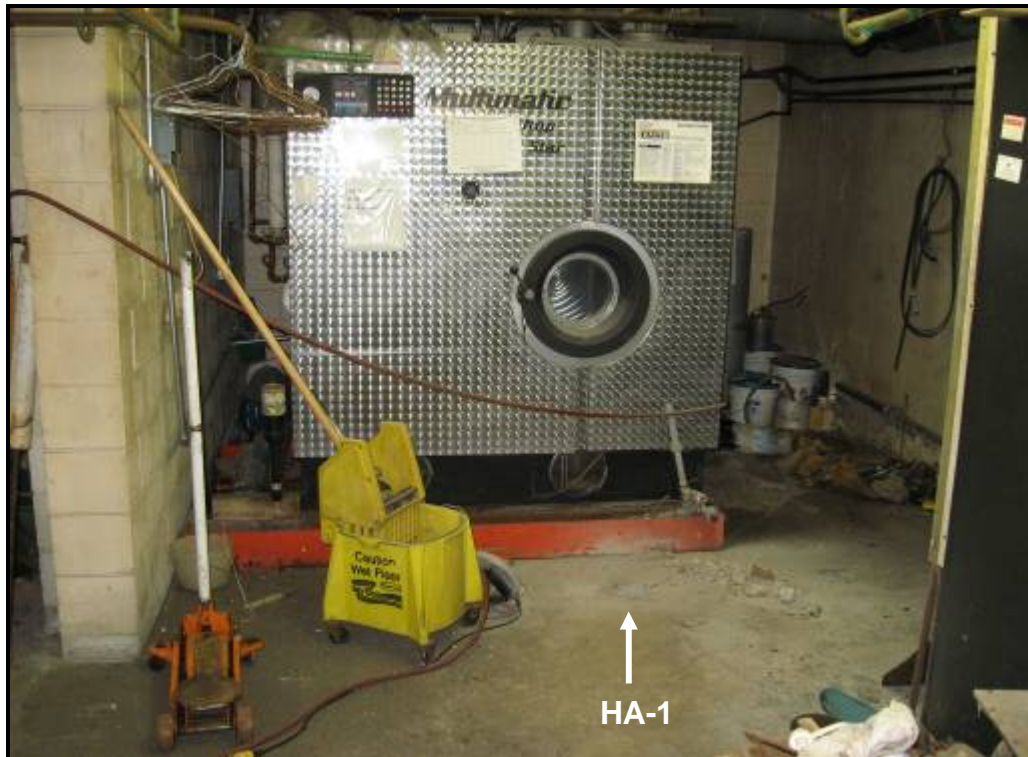
1) View of the location of soil boring HA-1 adjacent to the existing dry cleaning machine
