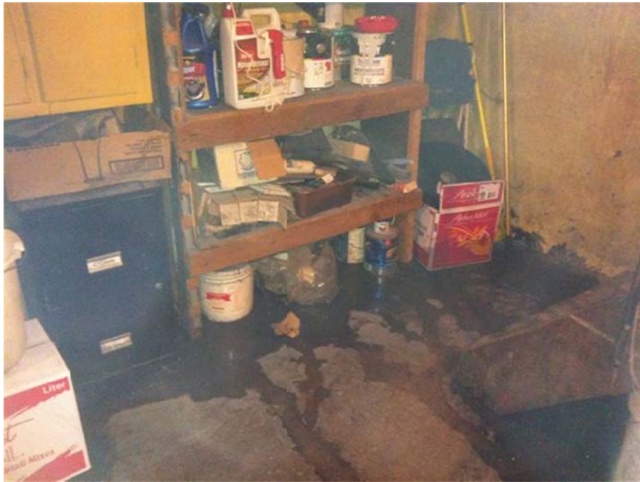
Photograph No.: 21 Photographer: Naren Babu Orientation: Southwest TDD Number: TO-05-11-03-0007 Contract: EP-S5-10-10, OTIE Date: April 18, 2011 Site Name & Location: Sandies Dry Cleaning Site, Little Chute, Outagamie County, Wisconsin. Subject: View of the adjoining wall inside the basement in Weenies Still Bar showing water seeping from the site source area due to cracks in the wall
