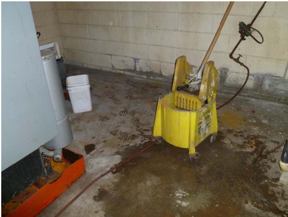
Photograph No.: 4 Photographer: Naren Babu Orientation: Southwest TDD Number: TO-05-11-03-0007 Contract: EP-S5-10-10, OTIE Date: April 7, 2011 Site Name & Location: Sandies Dry Cleaning Site, Little Chute, Outagamie County, Wisconsin. Subject: View of the bucket and mop from behind the dry cleaning machine in the wash room
