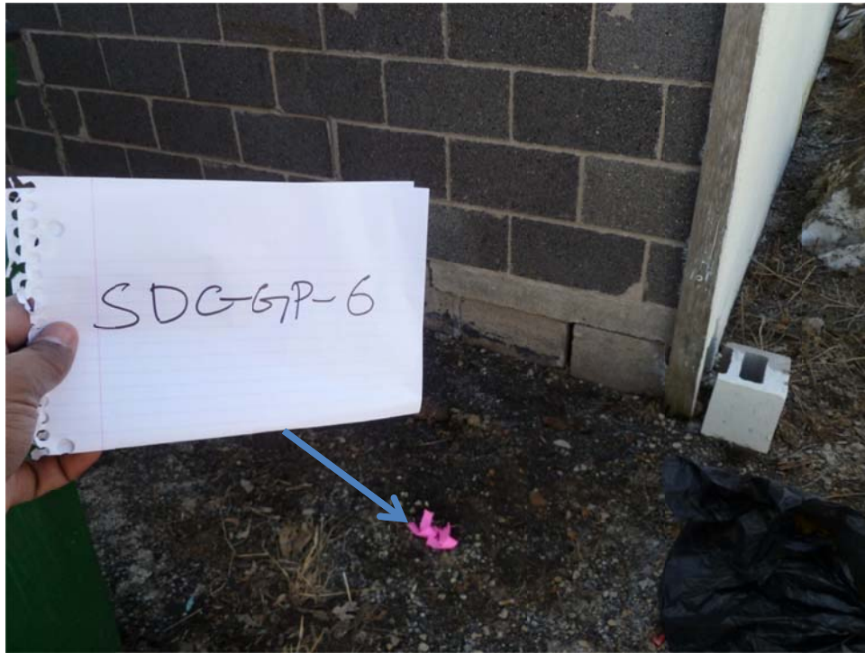
Photograph No.: 13 Photographer: Naren Babu Orientation: Southeast TDD Number: TO-05-11-03-0007 Contract: EP-S5-10-10, OTIE Date: April 7, 2011 Site Name & Location: Sandies Dry Cleaning Site, Little Chute, Outagamie County, Wisconsin. Subject: View of the location of soil boring SDC-GP-6 in the southwest side of the site
