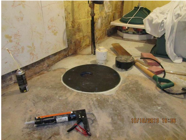
Photo 1: Looking northeast at installation of Pickup Point B
