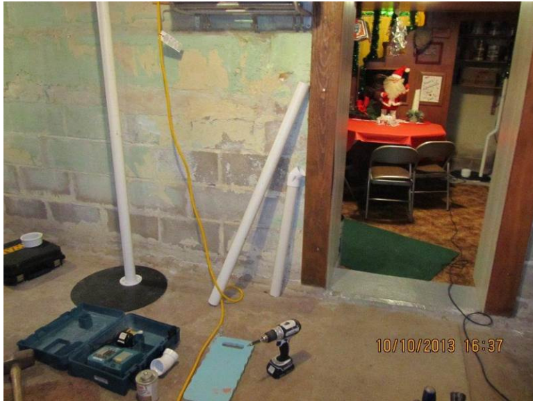
Photo 3: Looking southeast at Pickup Point A during construction
