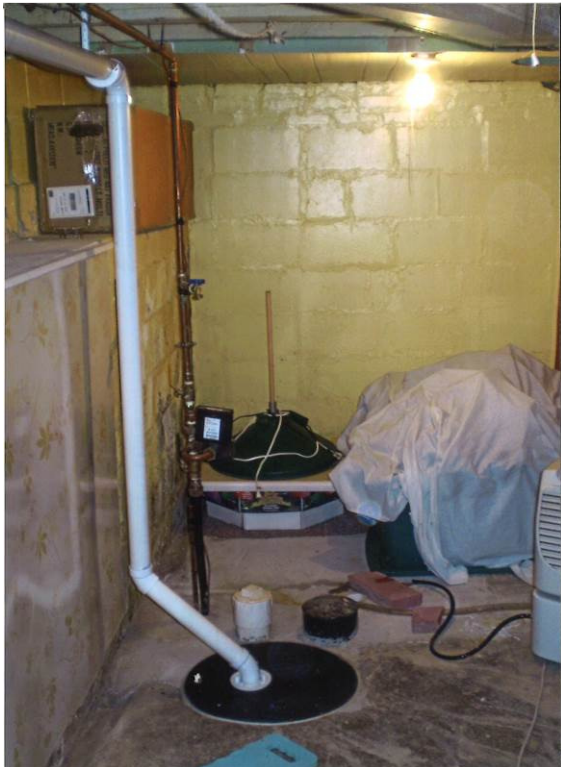
Photo 6: Looking east at completed Pickup Point B and PVC pipe
