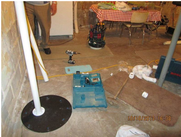
Photo 4: Looking west at Pickup Point A and drop pipe
