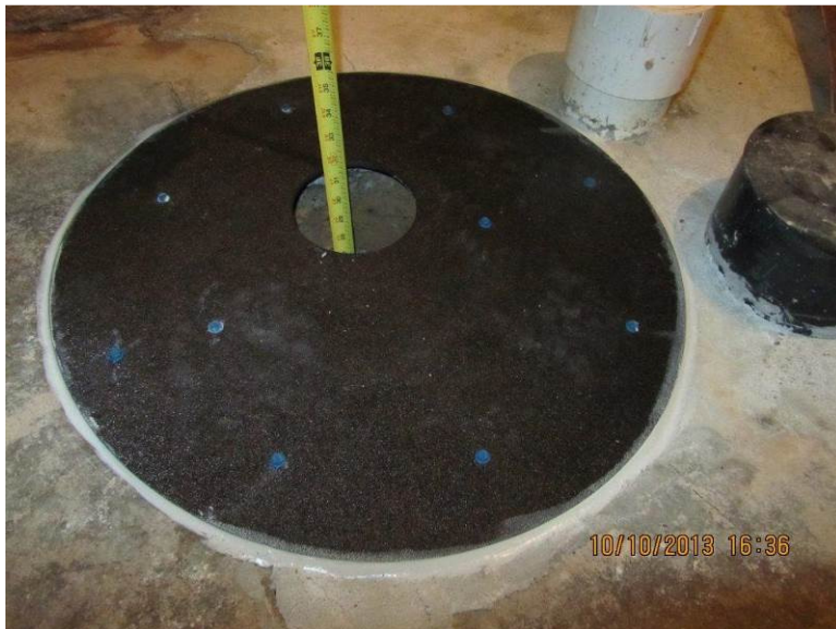
Photo 2: Pickup Point B cover and seal during installation
