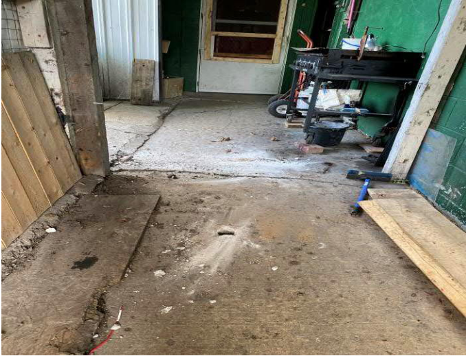
Photo #1 View of P-1 facing east towards Weenie's back entrance.
