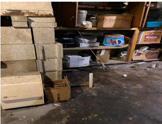
Photo #5 View of P-3 in Weenie's basement facing south.
