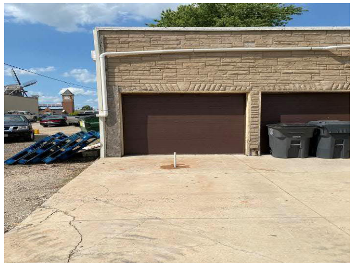
Photo #12 View P-8 in parking area adjacent to alley facing north.
