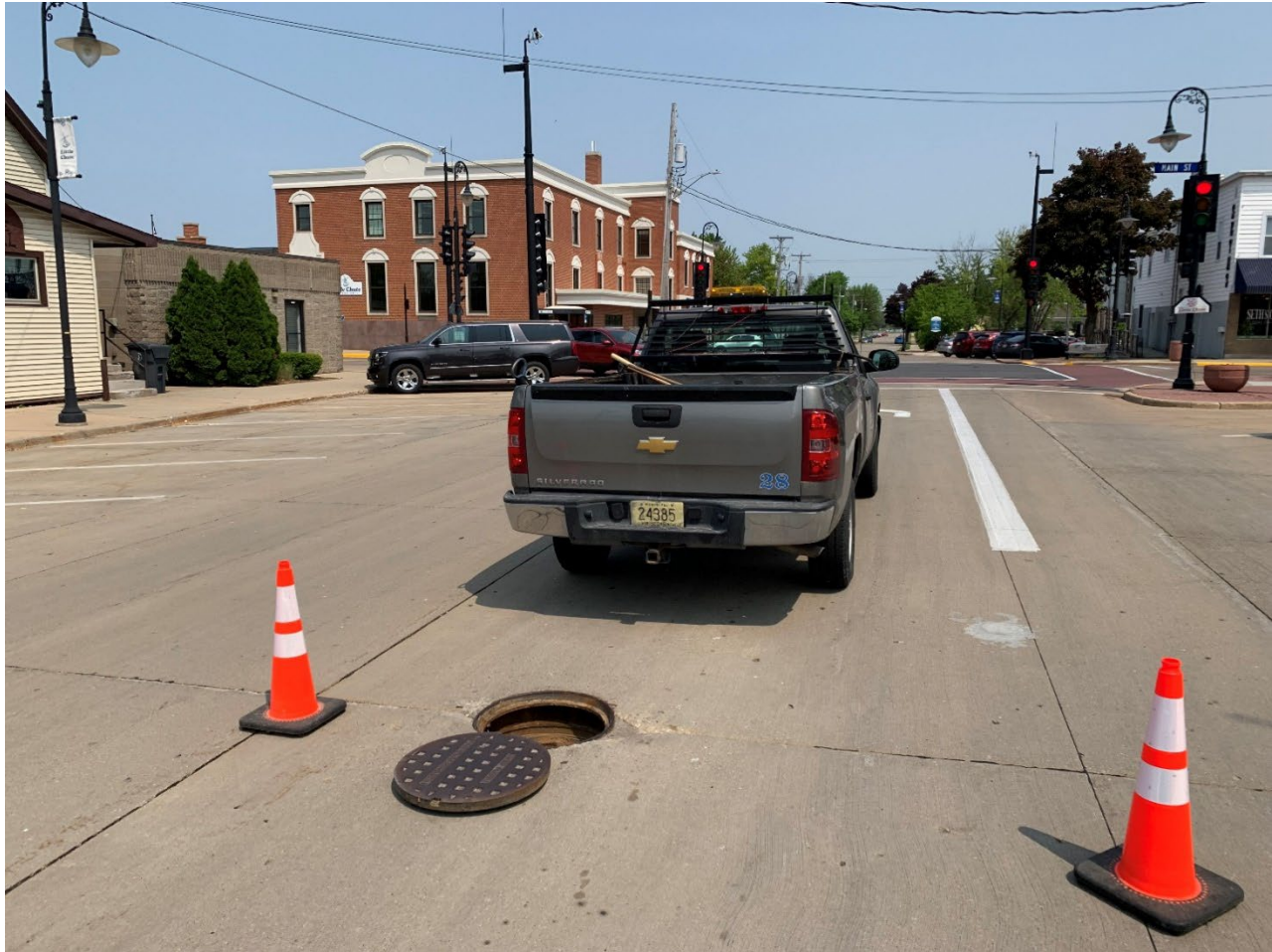
Photo 1: Looking north up Grand Ave with sanitary manhole “NMH0673/MH5” in the foreground. Traffic control measures provided by Village of Little Chute are shown as well.
