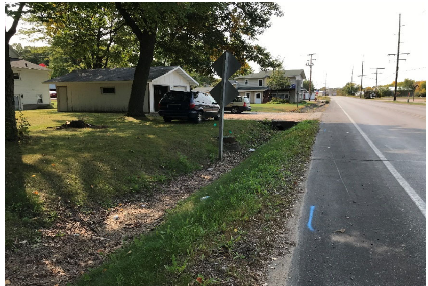
Sewer line on north side of Old Hwy 51 and manhole
