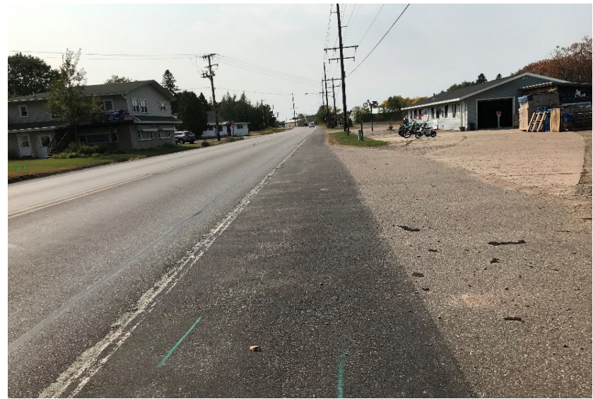
Sewer line on north side of Old Hwy 51, no manholes facing west from southwest corner of property
