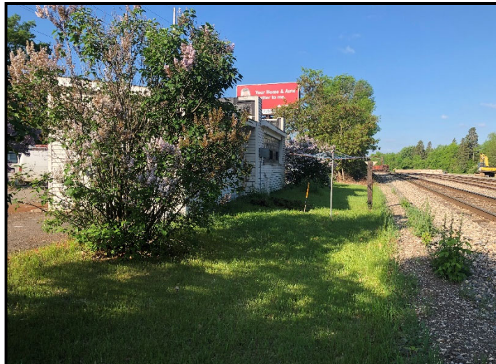
Rear of building and property line adjoining railroad right of way
