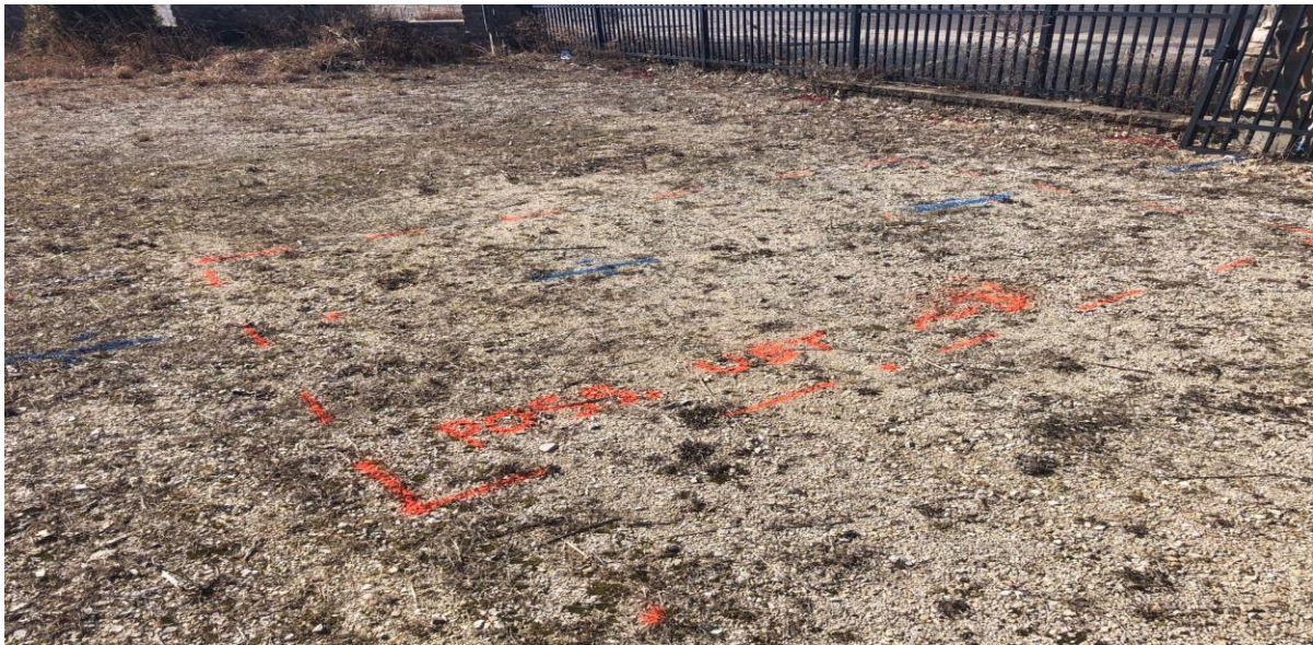
Site photo of the outline in orange of the possible UST and the blue markings of the water hose.
