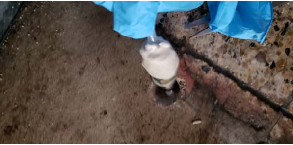
Installation of Modeling Clay Sealing in Vapor Sampling Port
