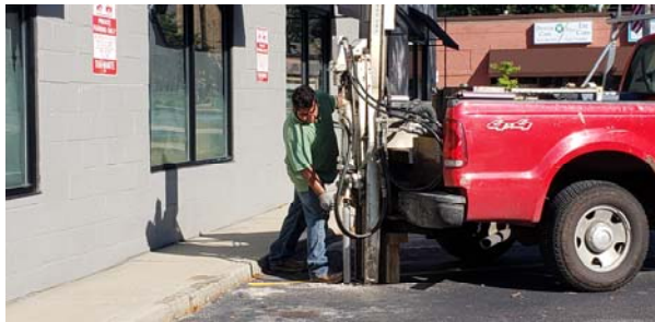
Installation of Soil Borings with Probing
