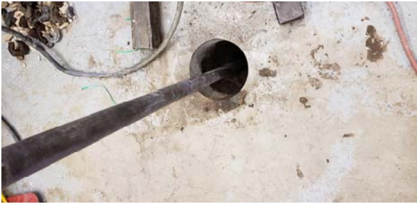
Boring with Probes
