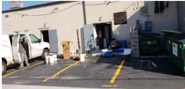
Back View (South Side) of the Drycleaning Store
