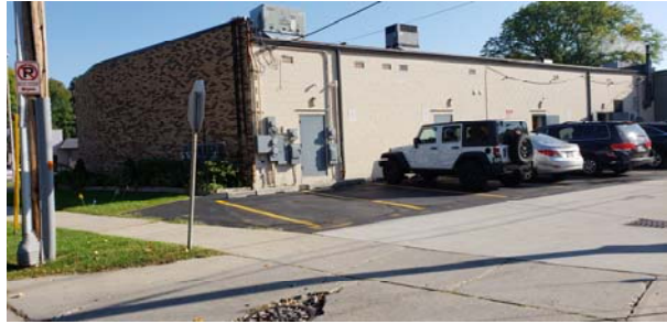
South and West Sides of the Strip Mall Building
