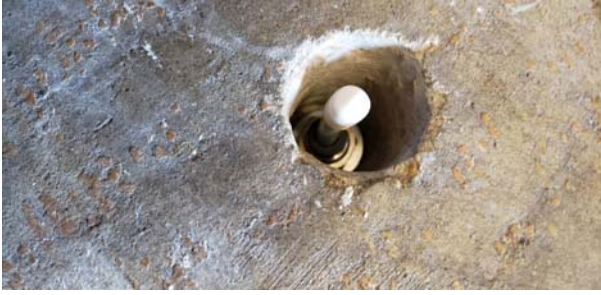
Sub-Slab Vapor Sampling Port Installation
