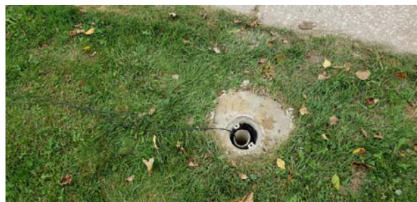
Connecting the Data Logger to Computer to Record the Water Level Change inside the Well after One Large Bailer of Water was Suddenly Removed from the Well
