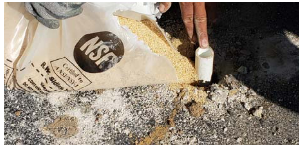
Installation of Monitoring Wells
