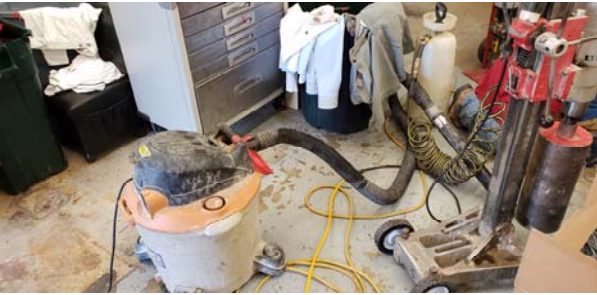
Concrete Coring for Soil Borings/Wells
