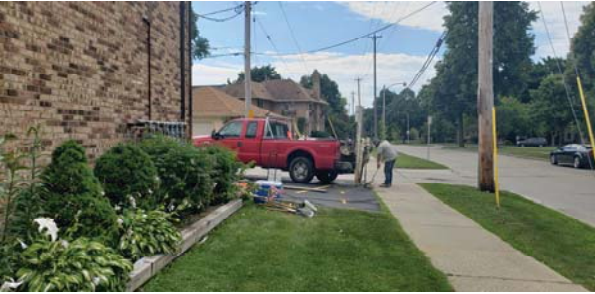
Soil Boring and Monitoring Well Installation
