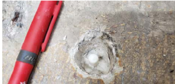
Finished New Soil Vapor Sampling Port
