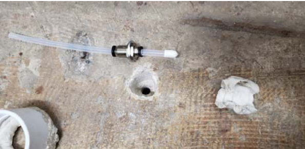
Installation of Soil Vapor Sampling Port on Concrete Floor
