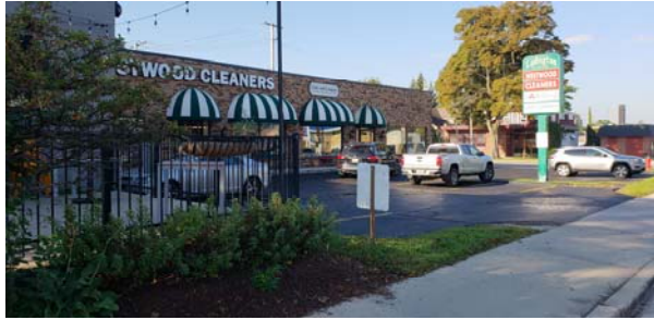
North Side of the Strip Mall Building
