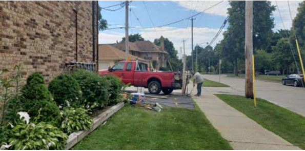
Soil Boring and Monitoring Well Installation
