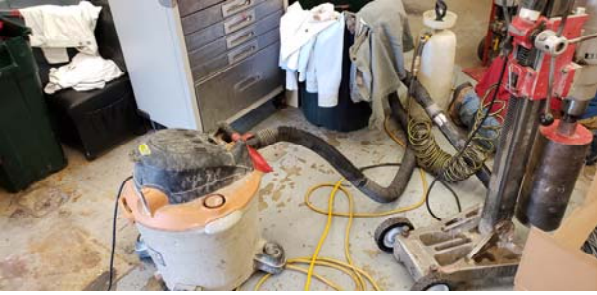
Concrete Coring for Soil Borings/Wells
