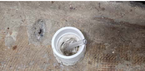
Water Dam Test for Vapor Port Leakage Check
