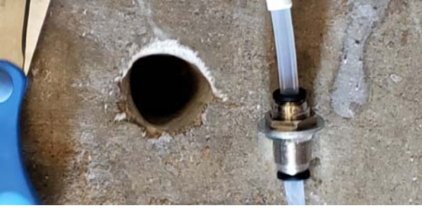
Sub-Slab Vapor Sampling Port Installation
