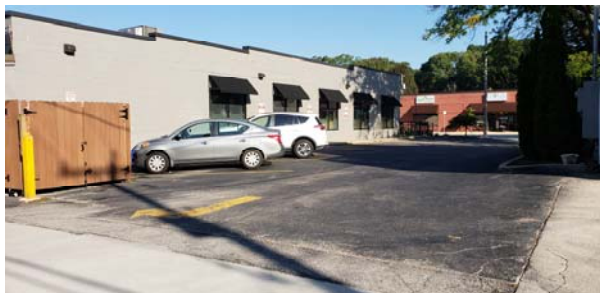
Parking Lot in the Neighboring Restaurant Property
