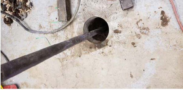
Boring with Probes
