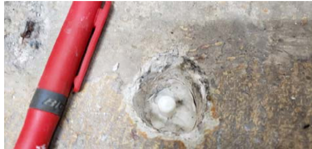
Finished New Soil Vapor Sampling Port
