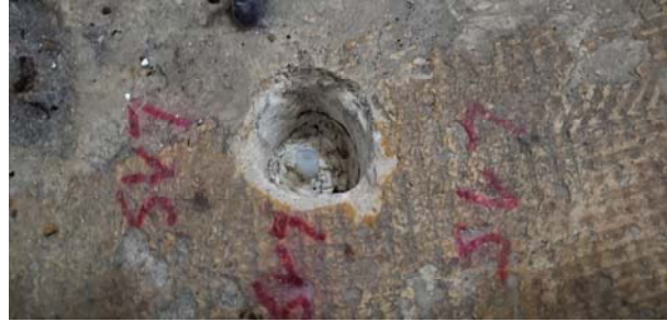
Sampling Port on Concrete Floor
