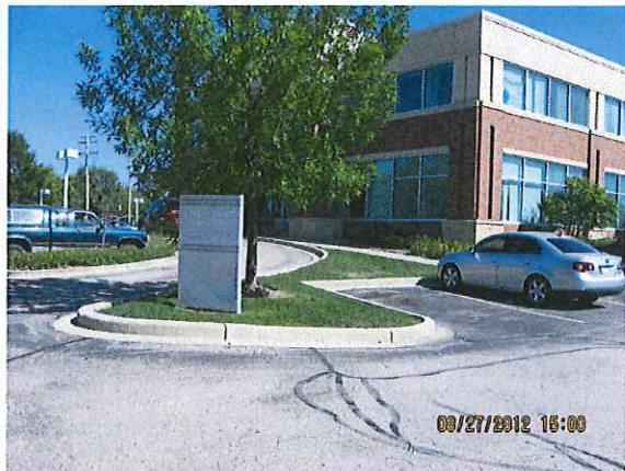
Looking ESE at drive-through at N end of medical building.
