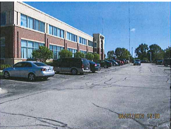
Looking S along W side of medical building.
