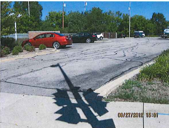
Looking ENE along N driveway into facility.
