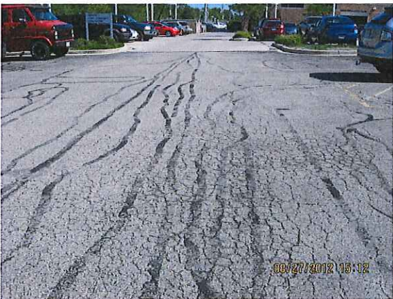
Looking S along pavement on E (back) side of facility.
