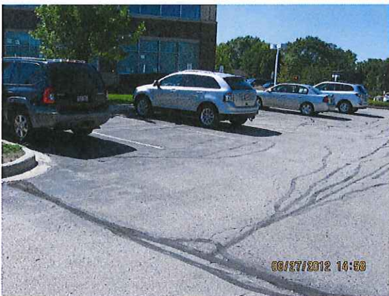
Looking NW at parking area E of medical building.
