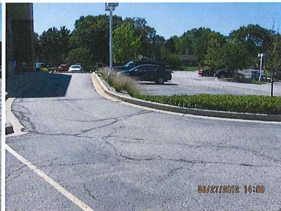
Looking W along drive-through at N end of medical building.
