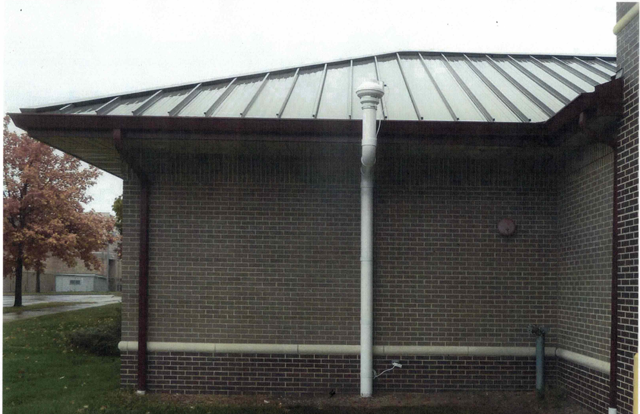
Proposed Exterior Vertical Pipe and Earth Gas Fan for the Commercial Building
