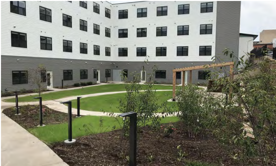
Photo 2: Courtyard area, looking SW, 10/2019.
