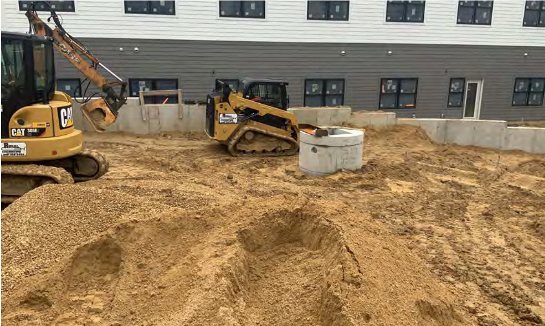
Photo 13: Plumbing work in courtyard area, 6/19/2019.
