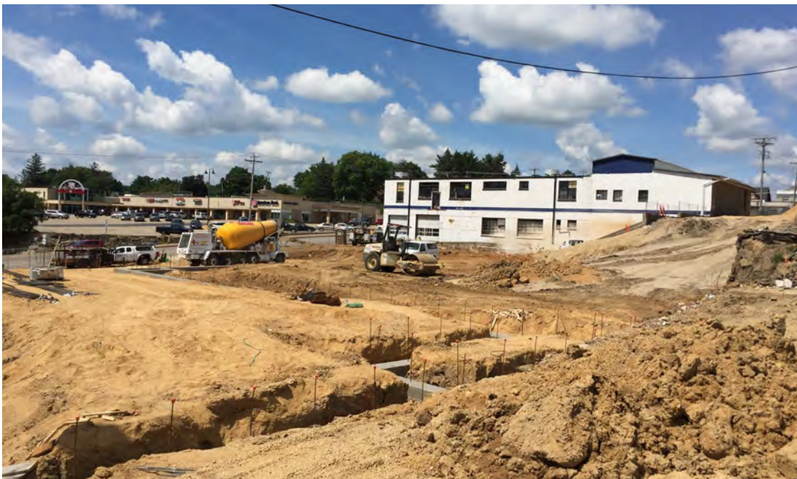
Photo 6: Foundation construction, looking SW towards E. Pine Street, 7/18/2018.
