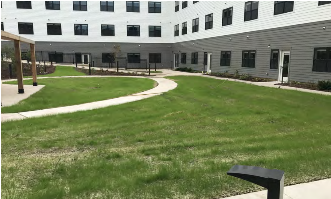
Photo 1: Courtyard area, looking E, 10/2019.
