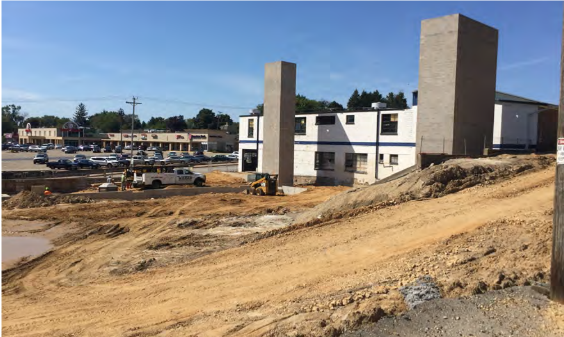
Photo 9: Building construction, looking SW towards E. Pine Street, 9/11/2018.
