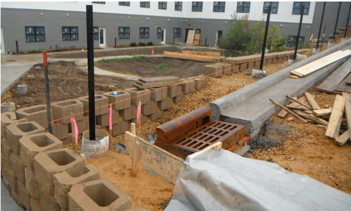
Photo 14: Backfill around retaining wall in courtyard, looking SW, 08/12/2019.
