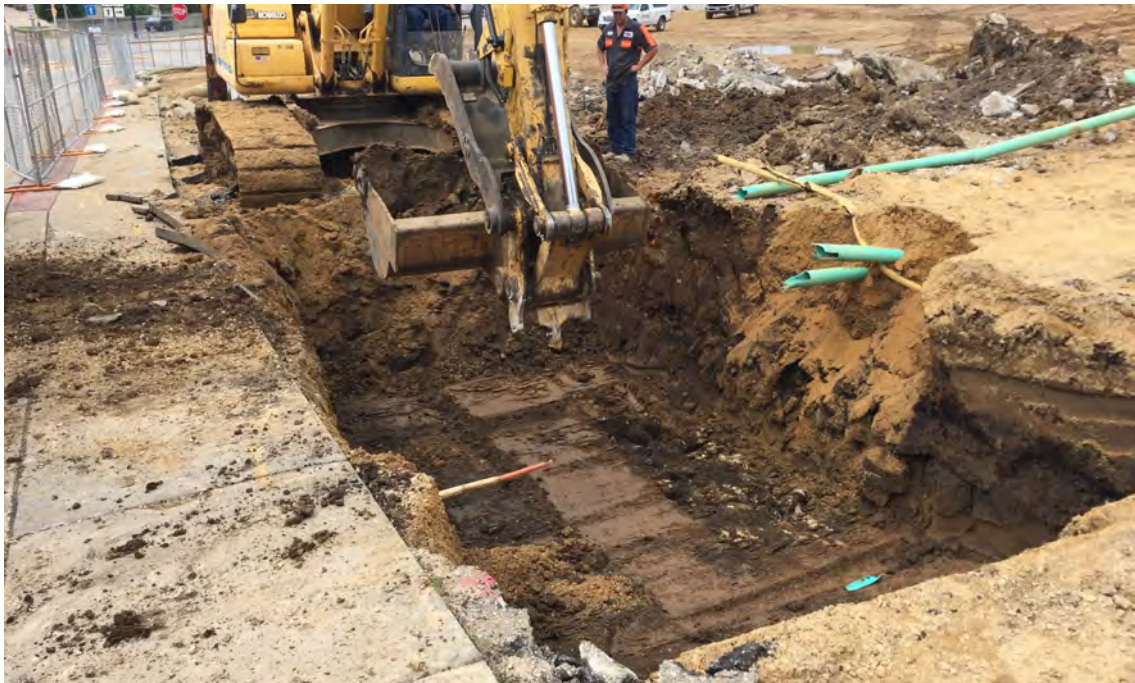
Photo 2: Targeted remedial excavation, looking S along N. Water St., 6/27/2018.
