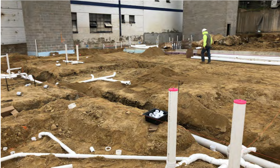
Photo 11: Plumbing work within building footprint, looking NW, 9/28/2018.
