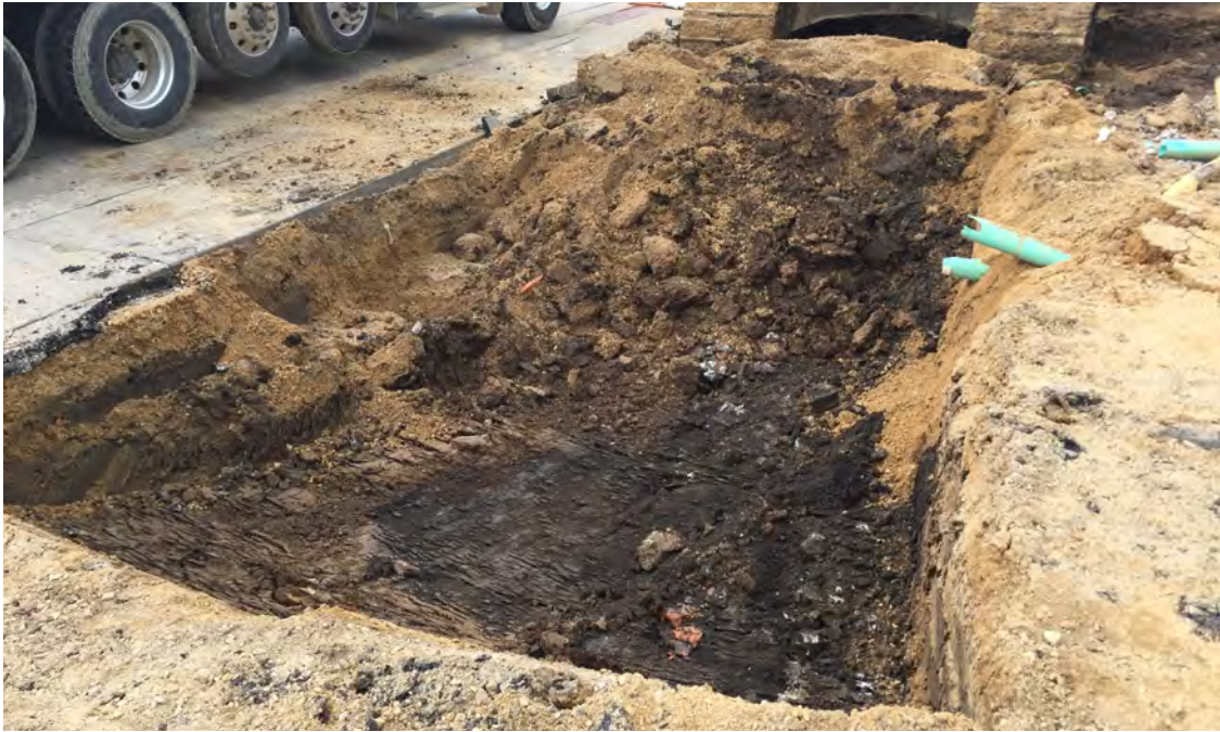
Photo 1: Targeted remedial excavation, looking S along N. Water Street, 6/27/2018.
