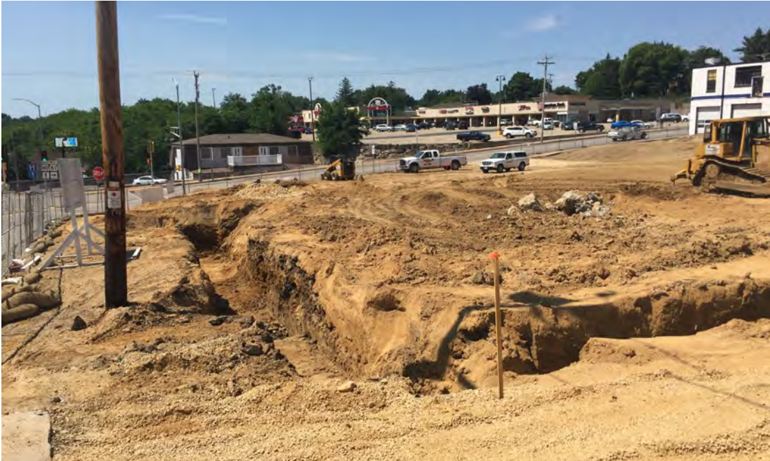
Photo 3: Initial foundation excavations, looking SW towards E. Pine Street, 7/9/2018.
