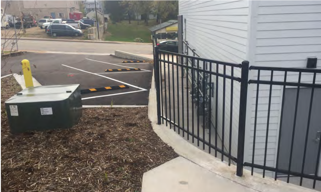
Photo 3: Looking E towards N. Water Street north of new building, 10/2019.
