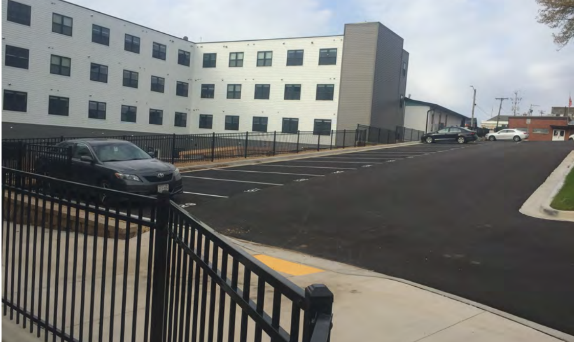
Photo 4: Looking west towards S. Oak Street area north of courtyard, 10/2019.
