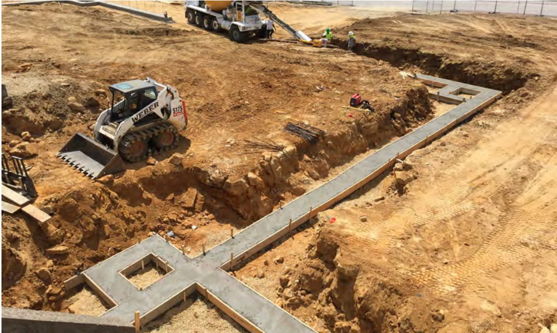
Photo 7: Foundation construction, looking SW towards E. Pine Street, 7/18/2018.
