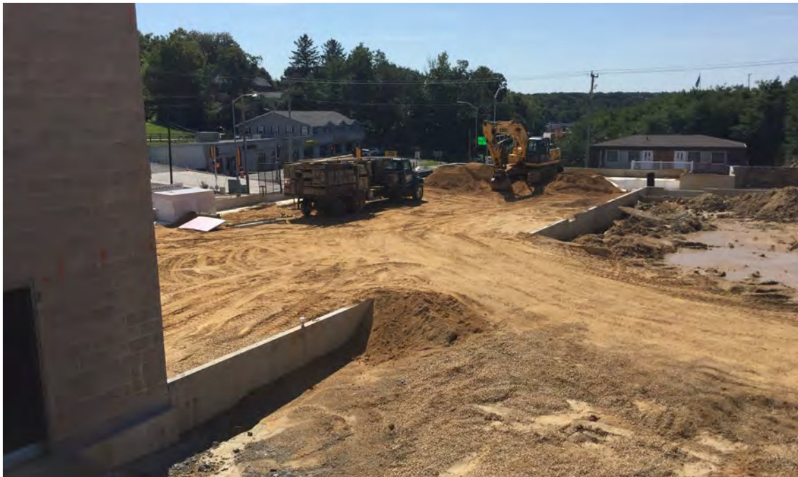
Photo 8: Building construction, looking SE towards E. Pine Street, 9/11/2018.
