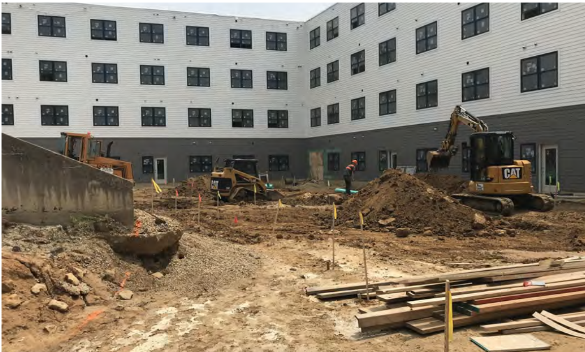
Photo 12: Exterior plumbing work, looking SE, 6/03/2019.
