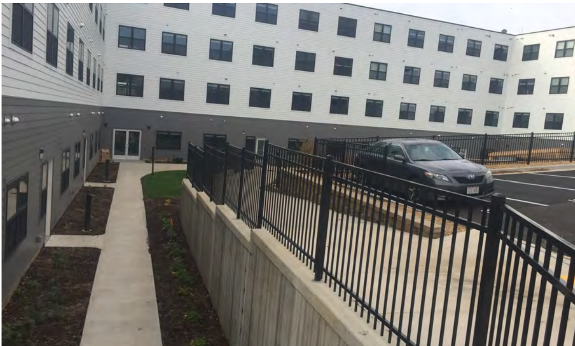
Photo 6: Looking S towards E. Pine Street, 10/2019.
