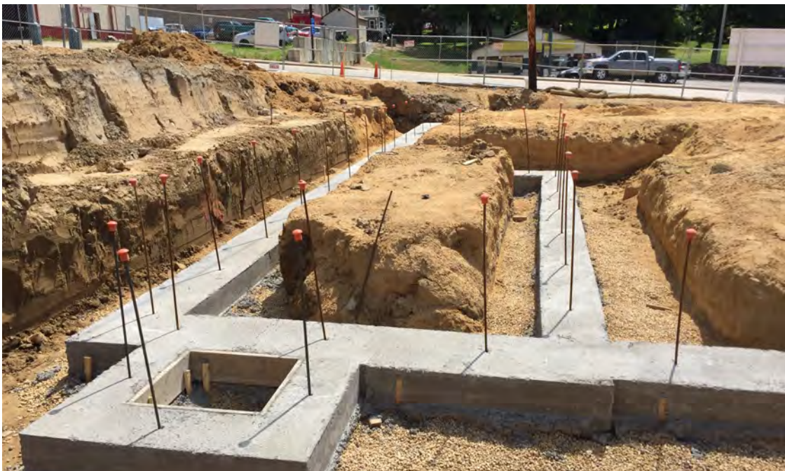
Photo 4: Foundation construction, looking S towards E. Pine Street, 7/18/2018.
