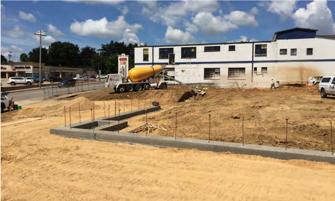
Photo 5: Foundation construction, looking west towards S. Oak Street, 7/18/2018.
