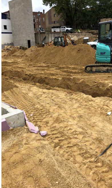
Photo 10: Plumbing work within building footprint, 9/28/2018.
