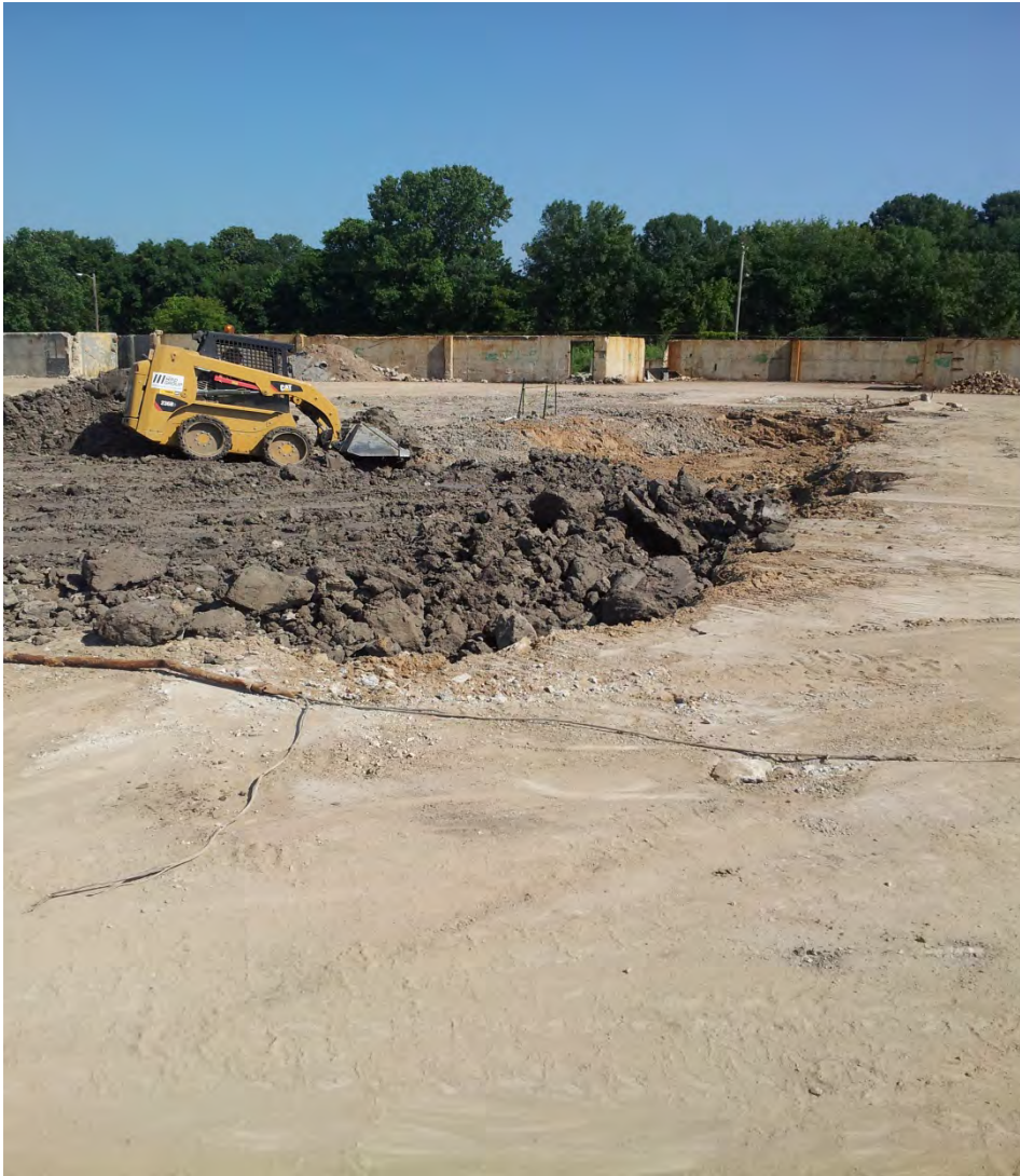
Photo Number: 9 Date of Photo: 7/15/13 Description: Backfilling Pit Excavations Creator: RJG
