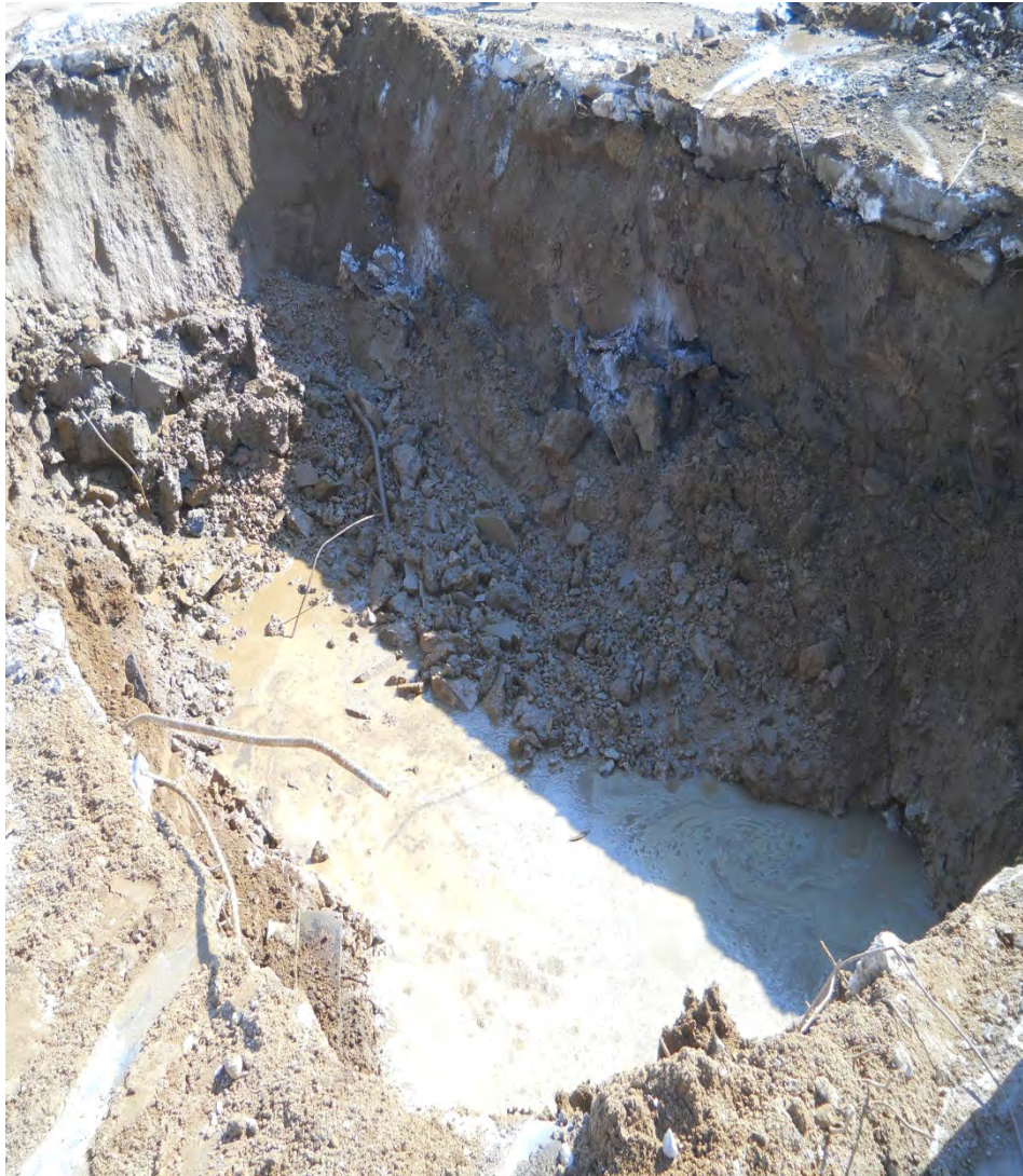
Photo Number: 8 Date of Photo: 7/10/13 Description: Removed Pit Excavation Creator: RJG
