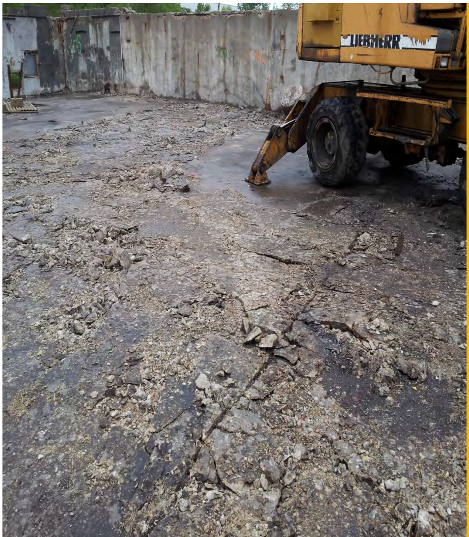
Photo Number: 2 Date of Photo: 5/22/13 Description: TSCA Floor Breaking Creator: RJG
