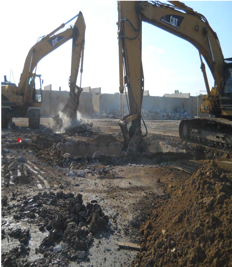
Photo Number: 7 Date of Photo: 7/10/13 Description: Ladle Pit Removal Creator: RJG
