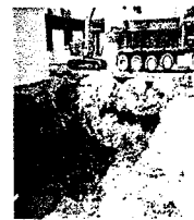
CONTAMINATED SOIL EXCAVATIONS
