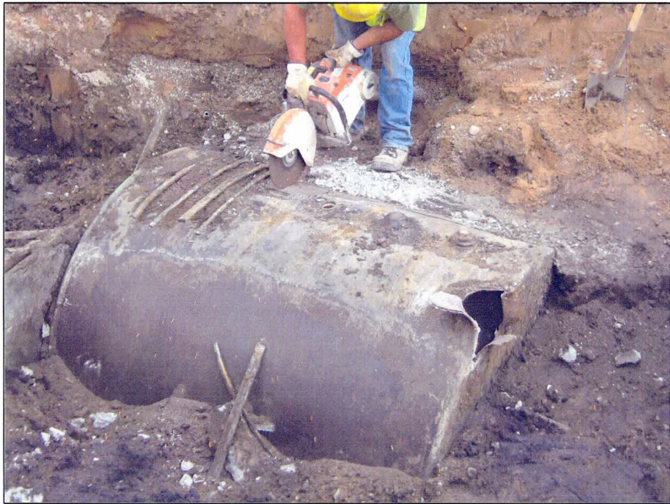
Photo 3 – Cutting Open of UST.
