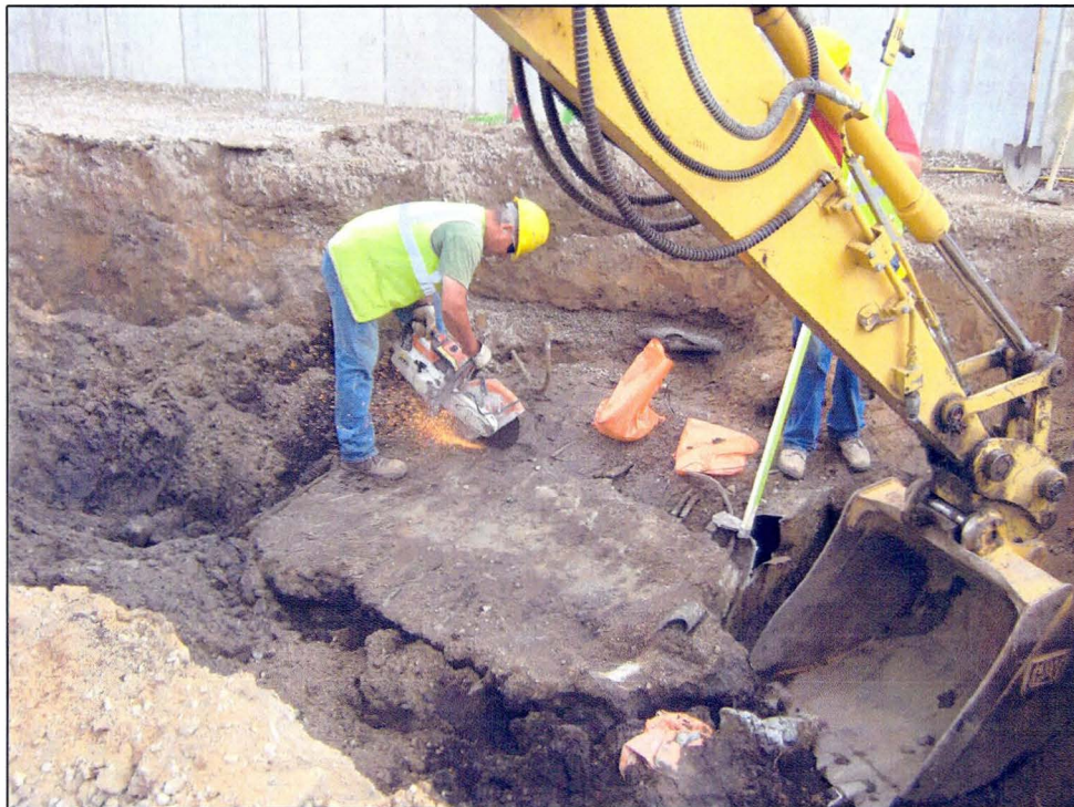
Photo 2 – Uncovering of the UST, Looking North.
