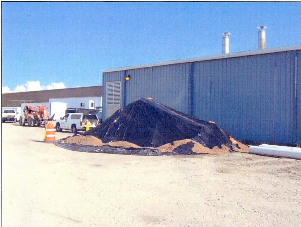
Photo 8 – Covered Soil Stockpile.
