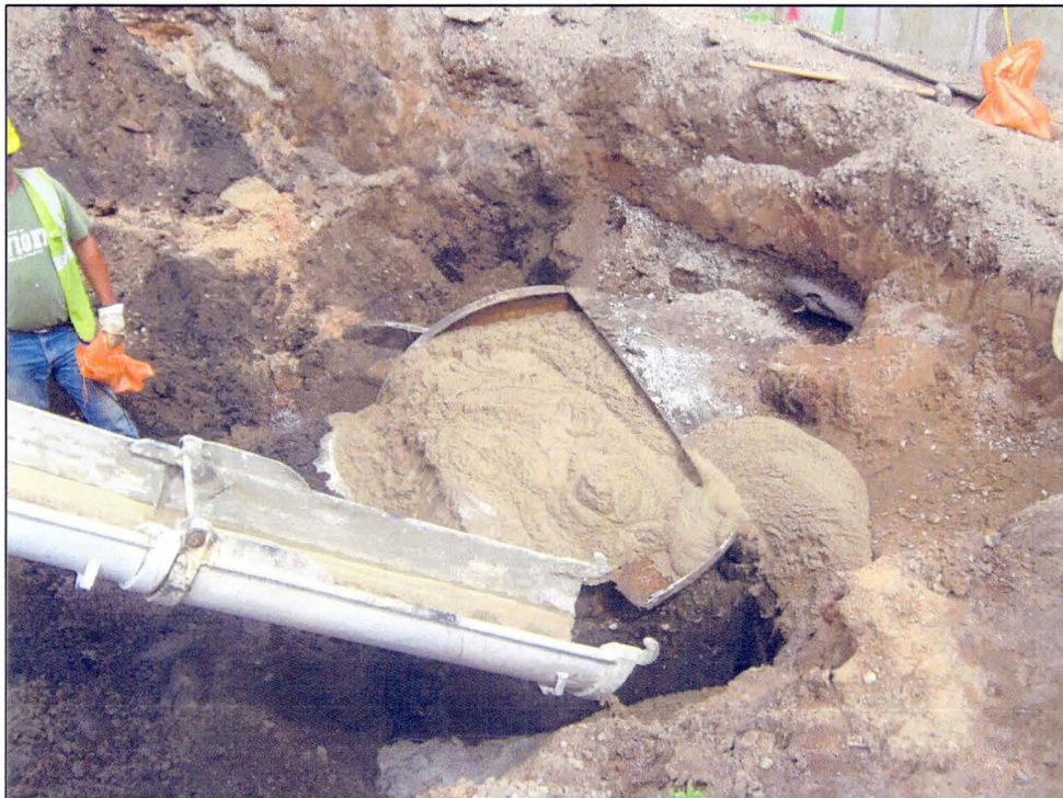
Photo 6 – Abandonment of UST with Concrete Slurry.
