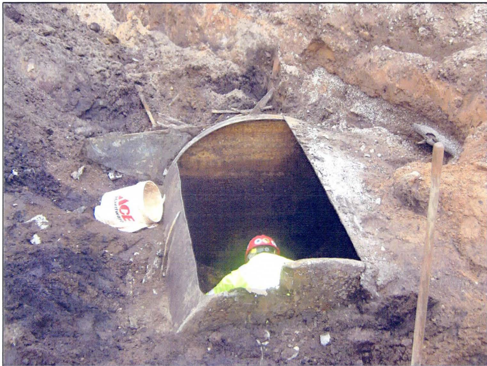
Photo 4 – Cleaning of UST.
