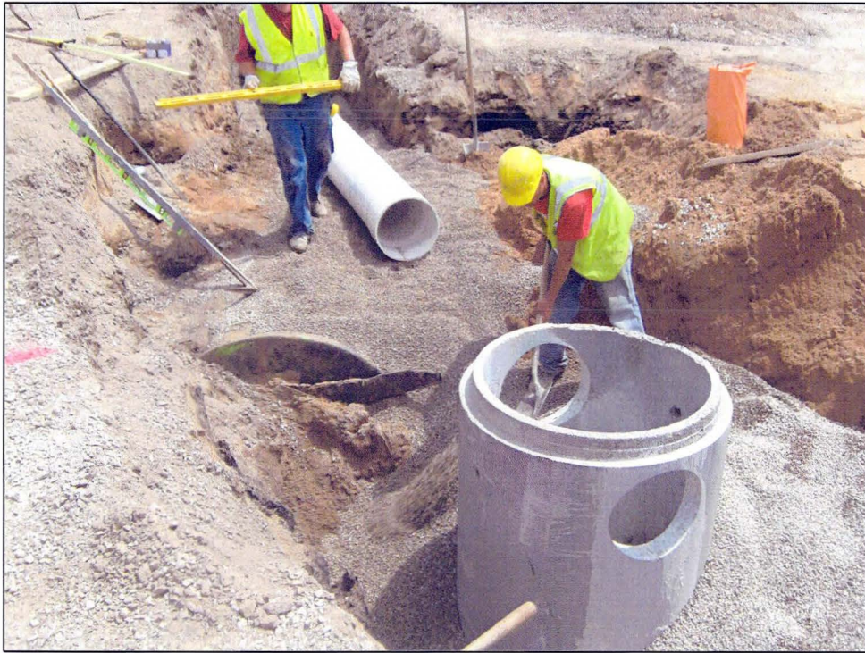
Photo 7 – Monitoring Well MW1, Located Top Right of Photo.
