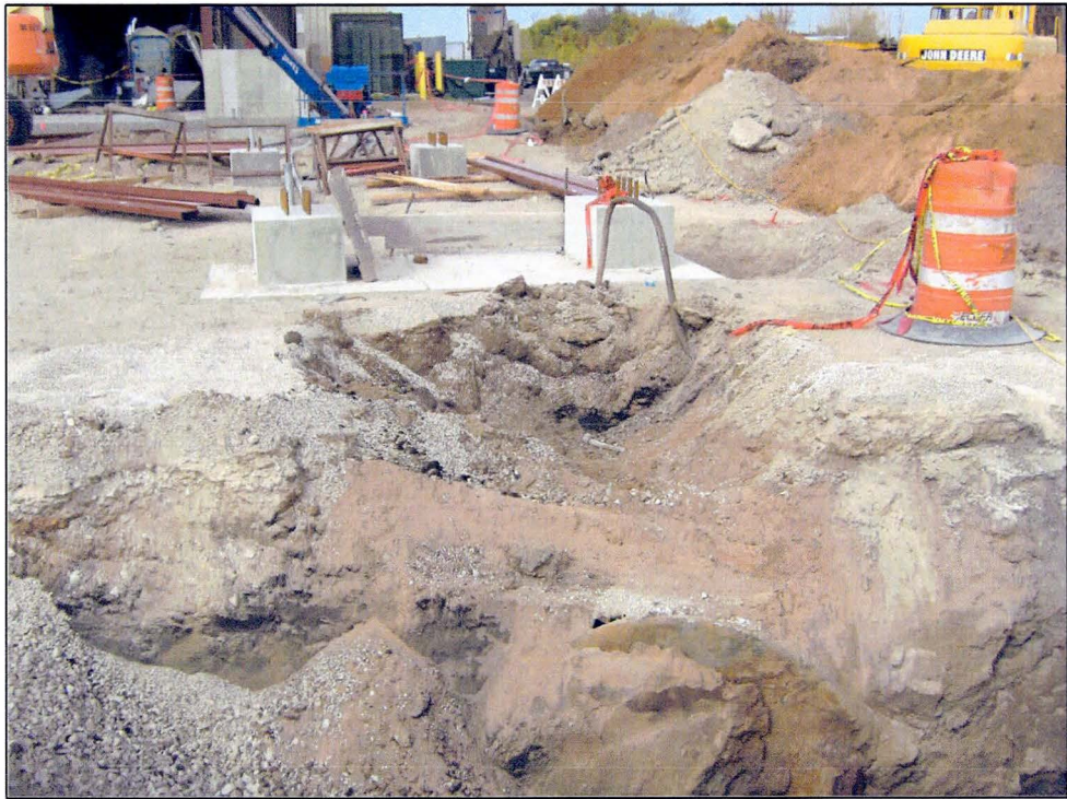
Photo 2 – Location of UST in Relation to Pile Cap.
