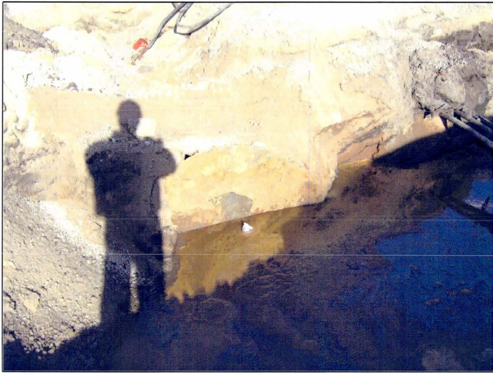
Photo 5 – Water in Excavation for Water Line Adjacent to UST.
