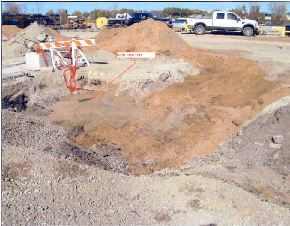
Photo 8 – UST Abandoned in Place with Concrete Slurry.
