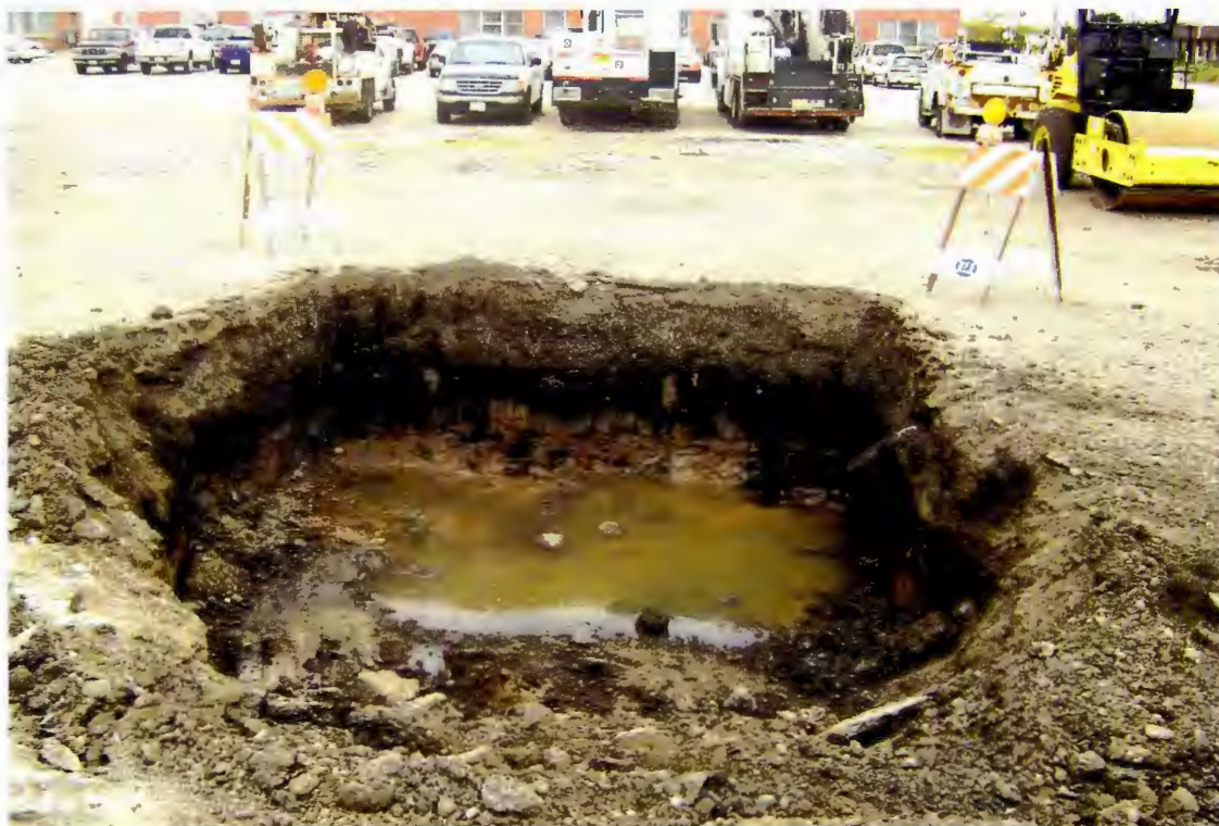
PHOTOGRAPH 4: View of Area 3 excavation looking east.
