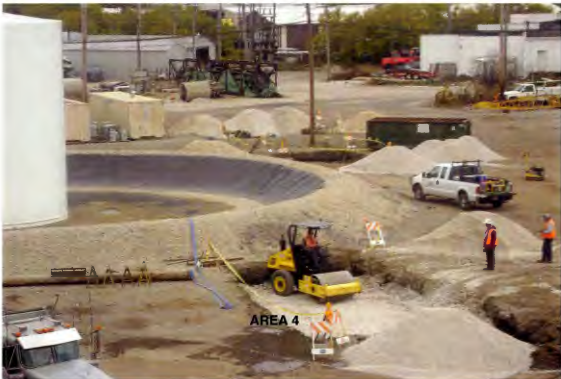
PHOTOGRAPH 12: View of Areas 1, 2, and 4 being backfilled.
