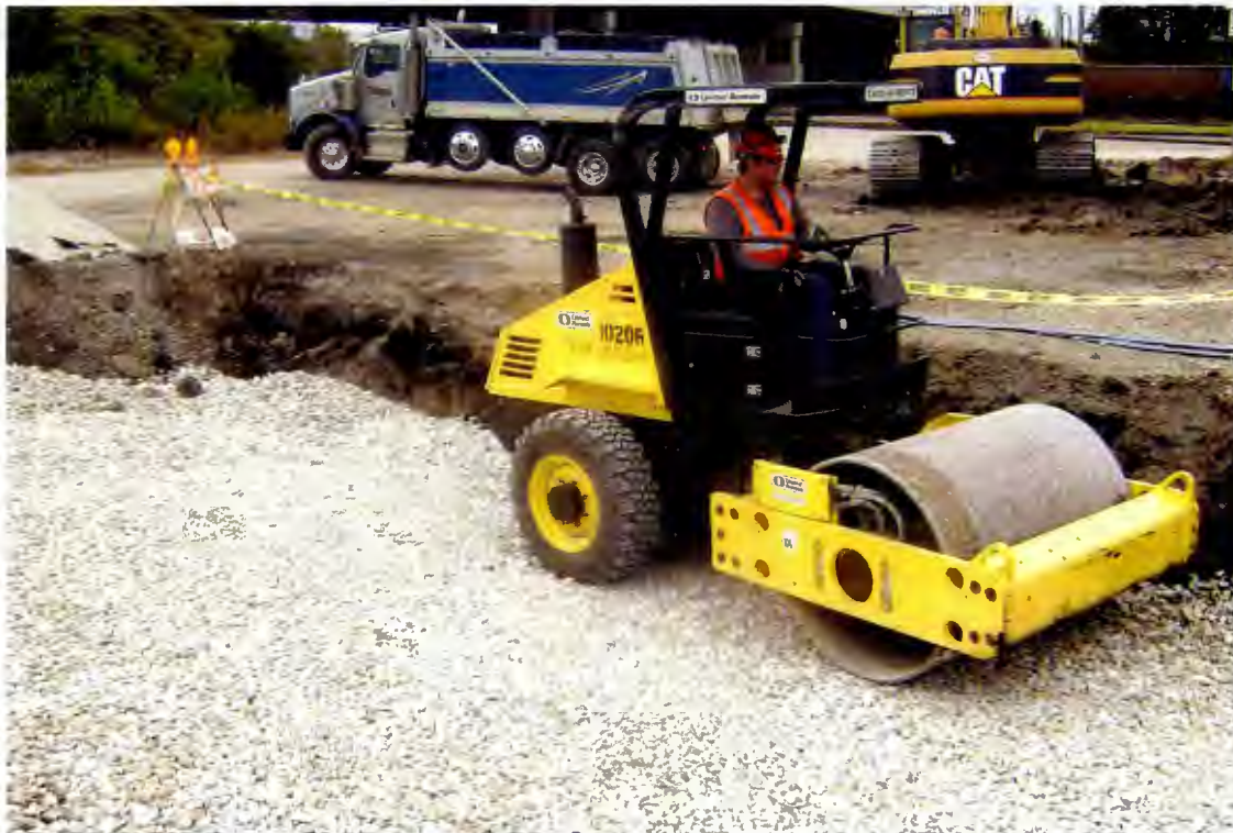
PHOTOGRAPH 7: View of area 4 excavation being backfilled.
