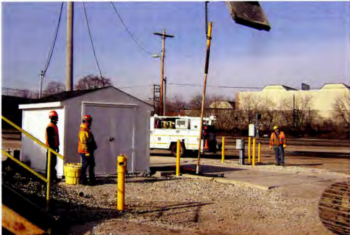
PHOTOGRAPH 1: MW-3 well abandonment.
