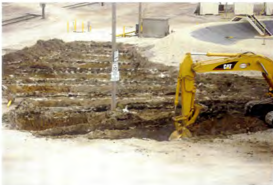
PHOTOGRAPH 10: View of Area 5 excavation in progress looking north. Concrete from former roundhouse shown.
