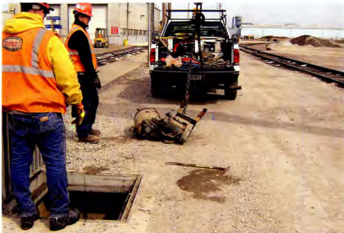
PHOTOGRAPH 6: Blower and knock out tank removed at VELR System #1.
