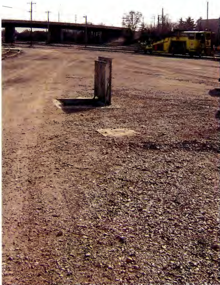
PHOTOGRAPH 3: VELR System #2 looking south, pre-decommissioning.
