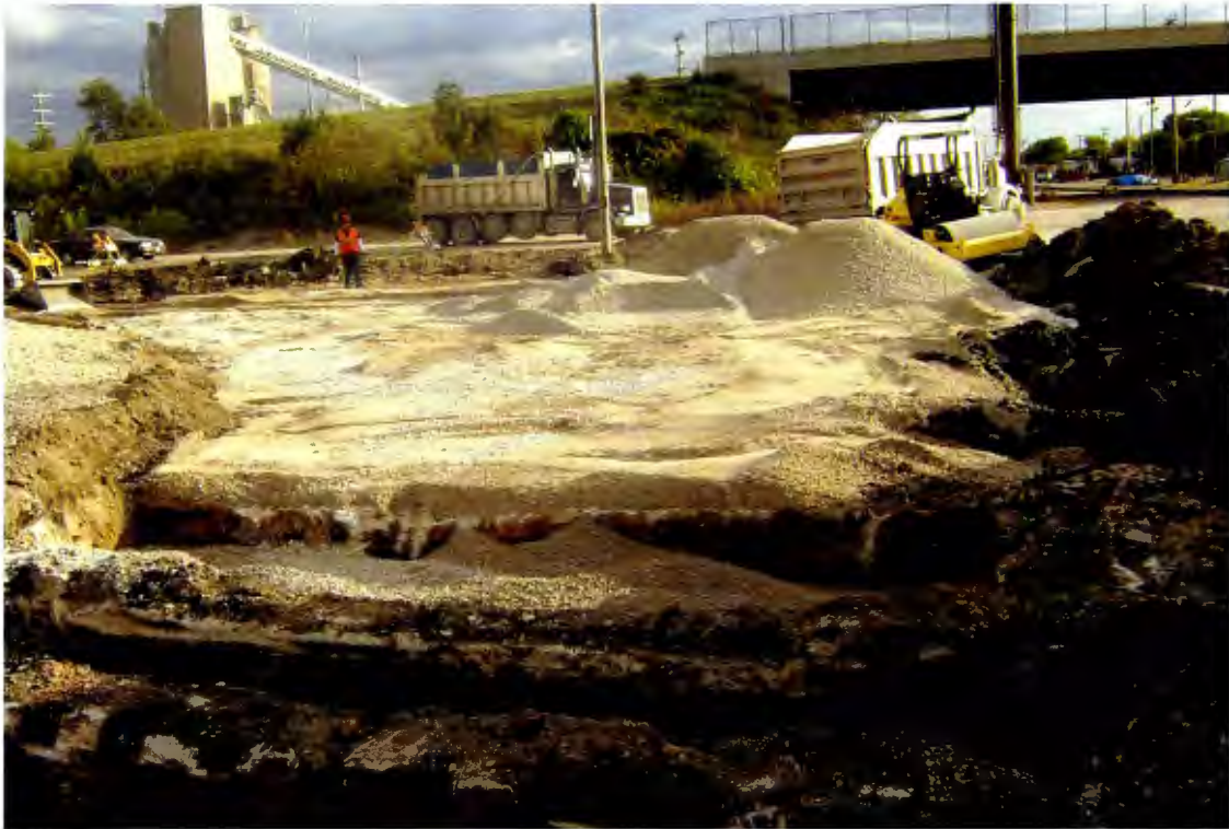
PHOTOGRAPH 11: View of Area 5 excavation being backfilled (looking south). Concrete from former roundhouse shown.
