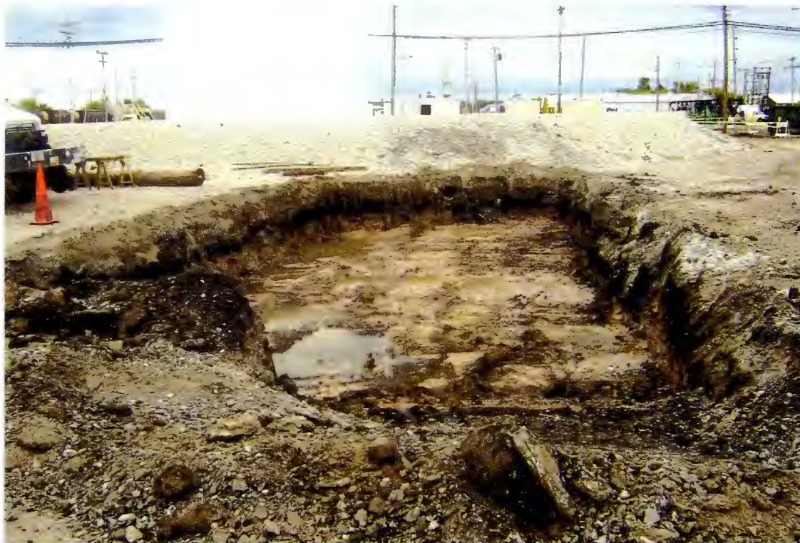
PHOTOGRAPH 5: View of Area 4 excavation looking north.
