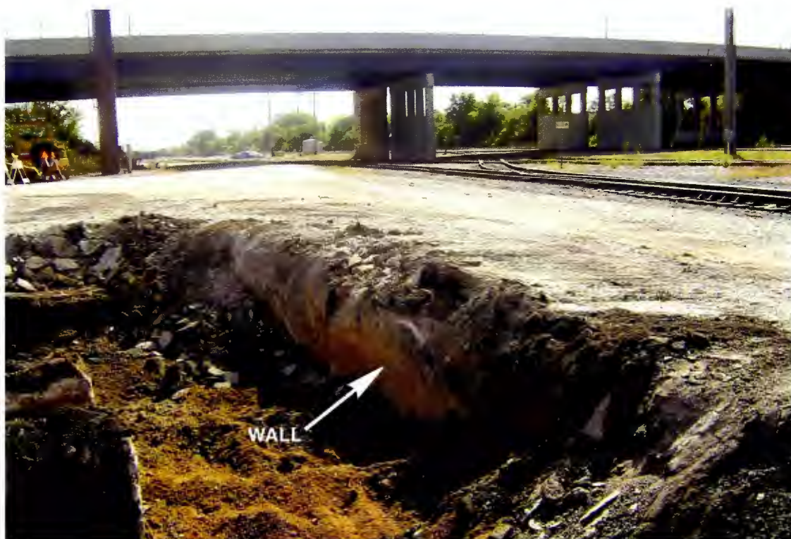
PHOTOGRAPH 8: View looking south at north south trending concrete wall extending to depth greater than 4 feet below land surface at Area 5 excavation.
