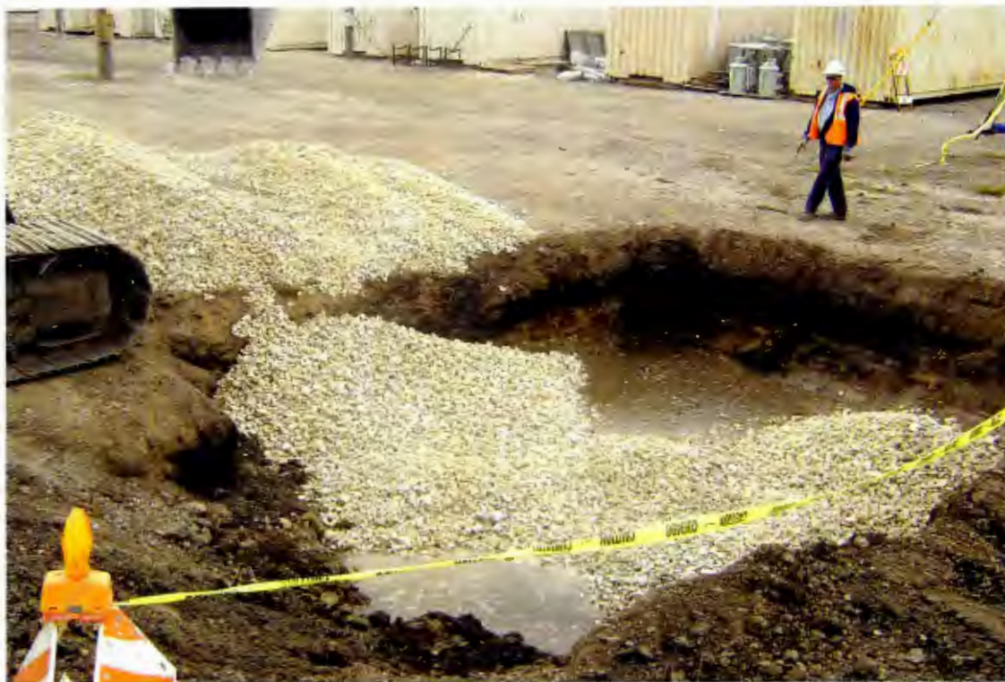
PHOTOGRAPH 3: View of Area 2 excavation being backfilled (looking north).
