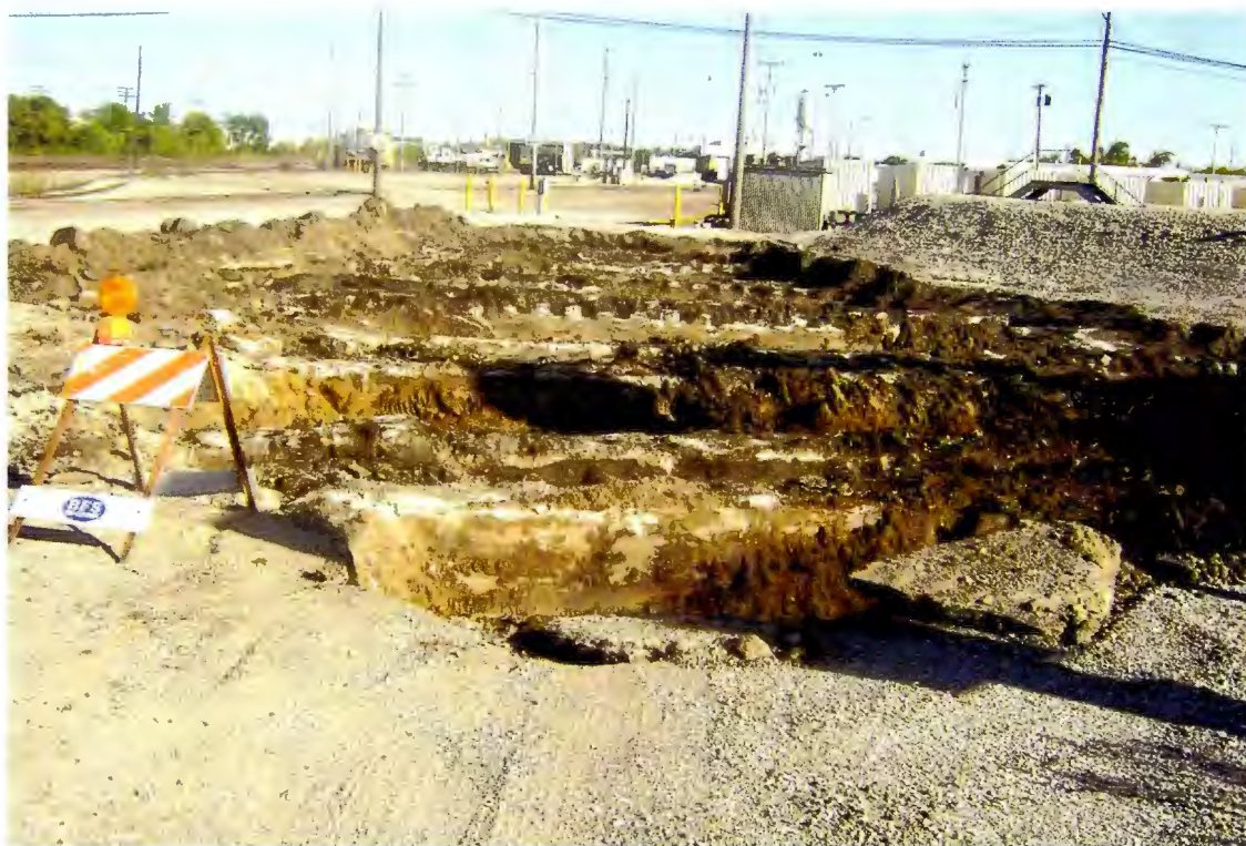
PHOTOGRAPH 9: View of Area 5 excavation looking north.
