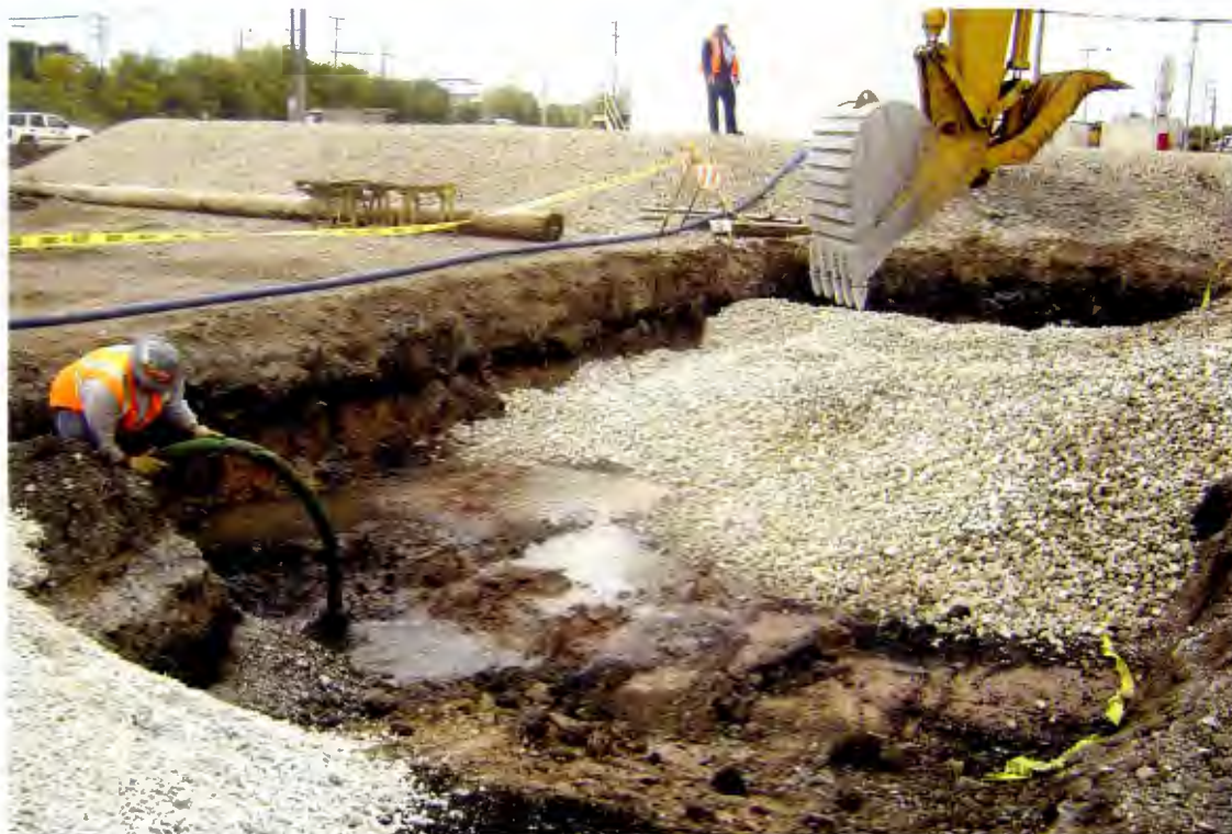
PHOTOGRAPH 6: View of Area 4 excavation being dewatered and backfilled (looking north).
