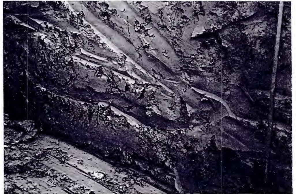
PHOTO #5 SIDE WALL OF EXCAVATION
