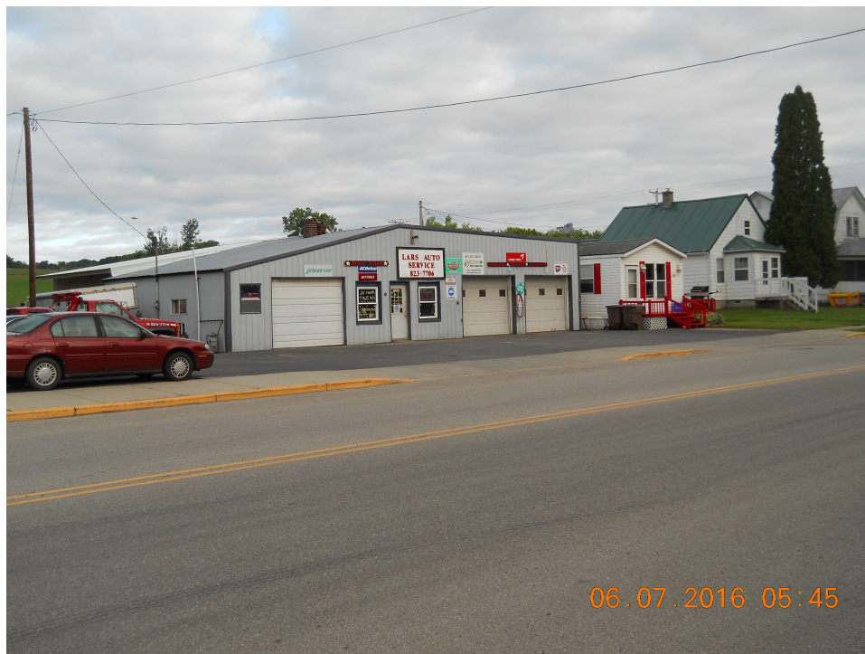
Photo 1: Looking northwest at service station building and asphalt lot.
