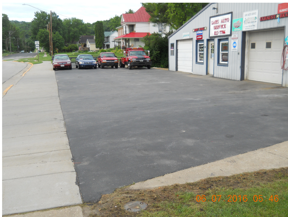
Photo 3: Looking south at asphalt cap to maintained (area of fmr UST systems).
