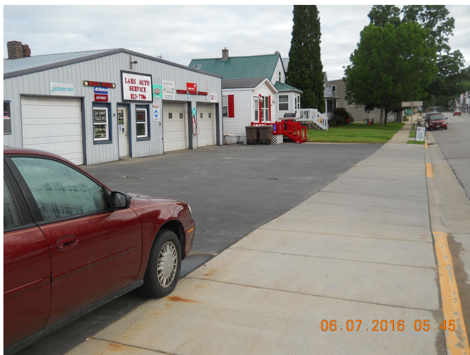
Photo 2: Looking north at asphalt cap to maintained (area of fmr UST systems).
