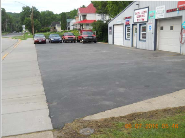
Title: Looking south at asphalt cap to maintained (area of fmr UST systems).
