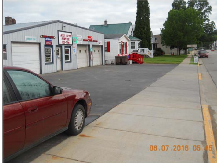
Title: Looking north at asphalt cap to maintained (area of fmr UST systems).
