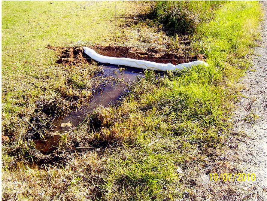
New Absorbents Placed
