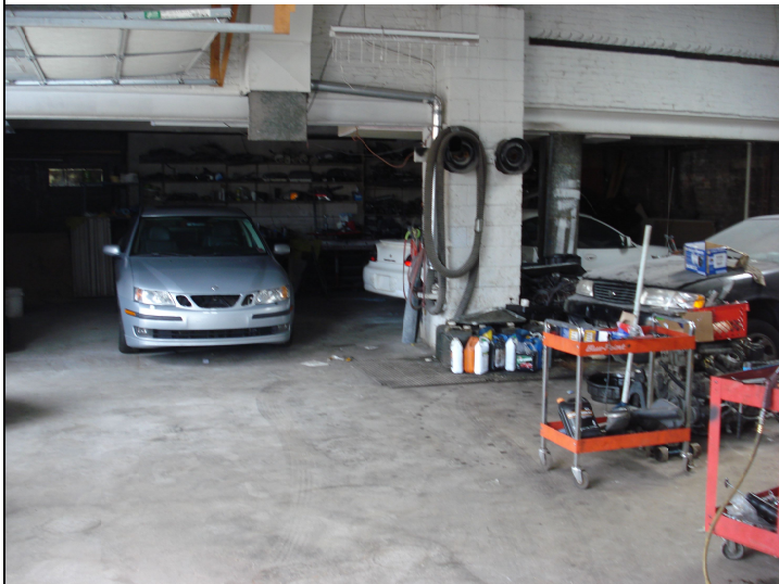
Title: Concrete Shop Floor
