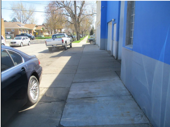
Title: East side concrete walk and apron facing south
