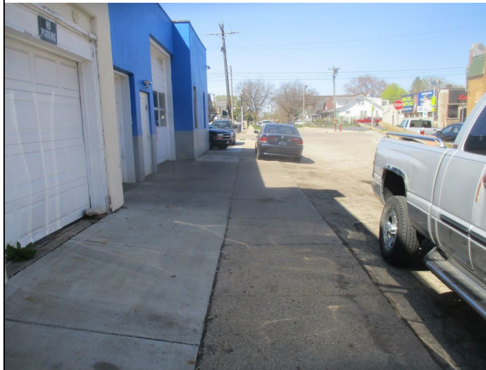
Title: East side concrete walk and apron facing north
