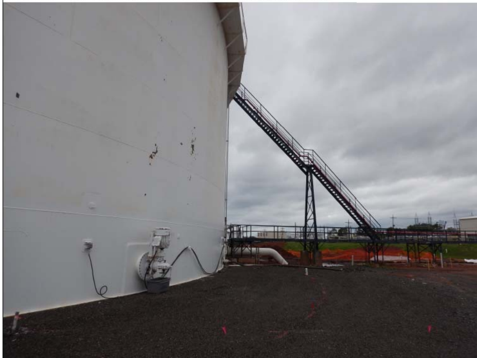
Title: Enbridge Energy Tank 22 looking NE
