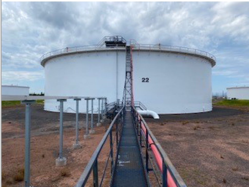
Title: South side of Tank 22. Photo taken facing northwest on 7/18/2022.
