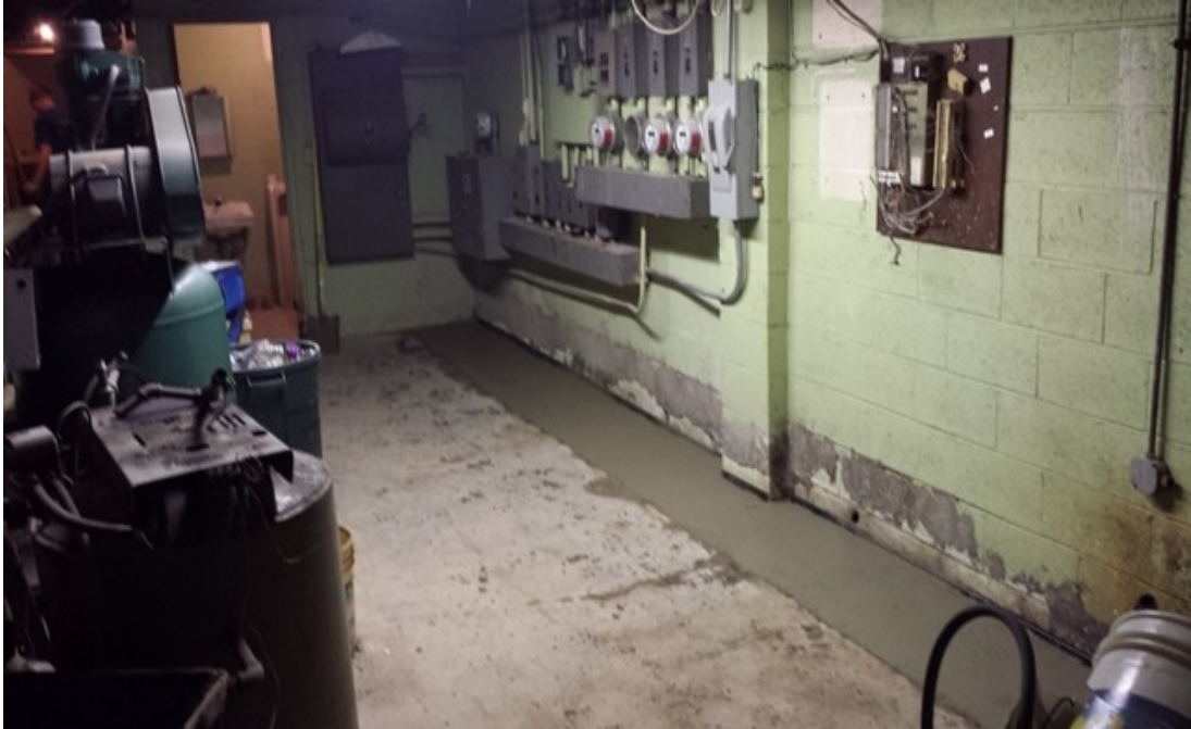
Above: Concrete restoration in basement along west wall.
