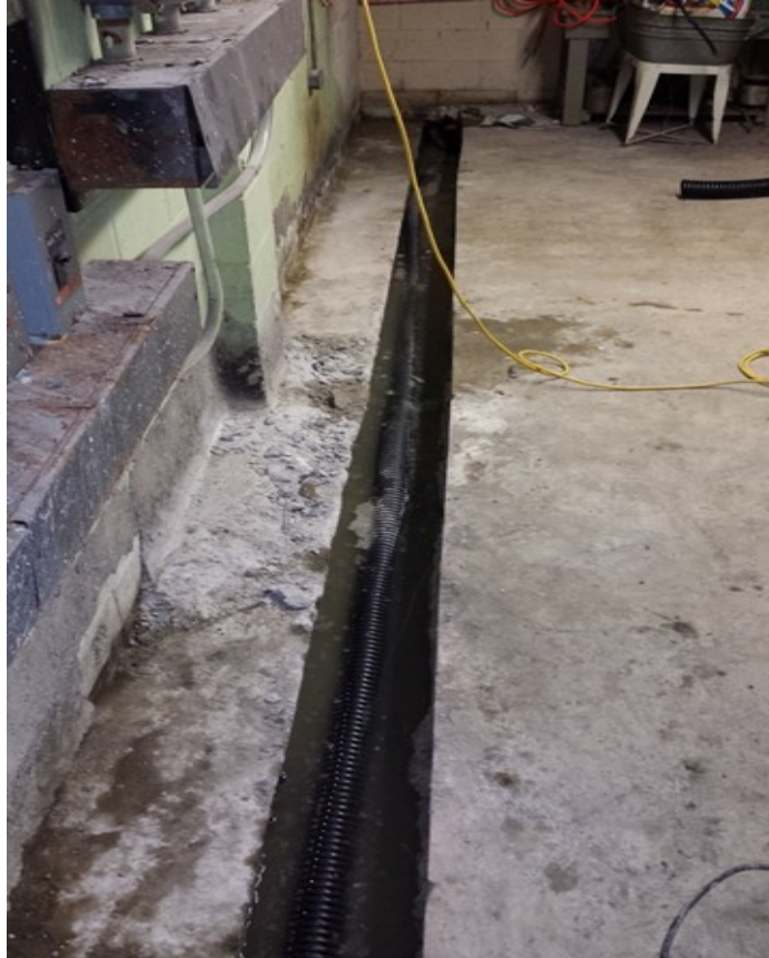
Below: 4-inch diameter drain pipe is set in basement trench along west foundation wall.
