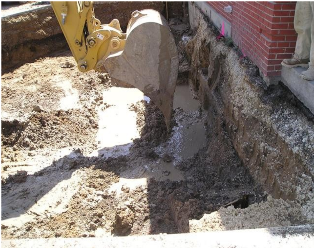
Below: Roof-drain storm laterals broken with water entering excavation following rain event.
