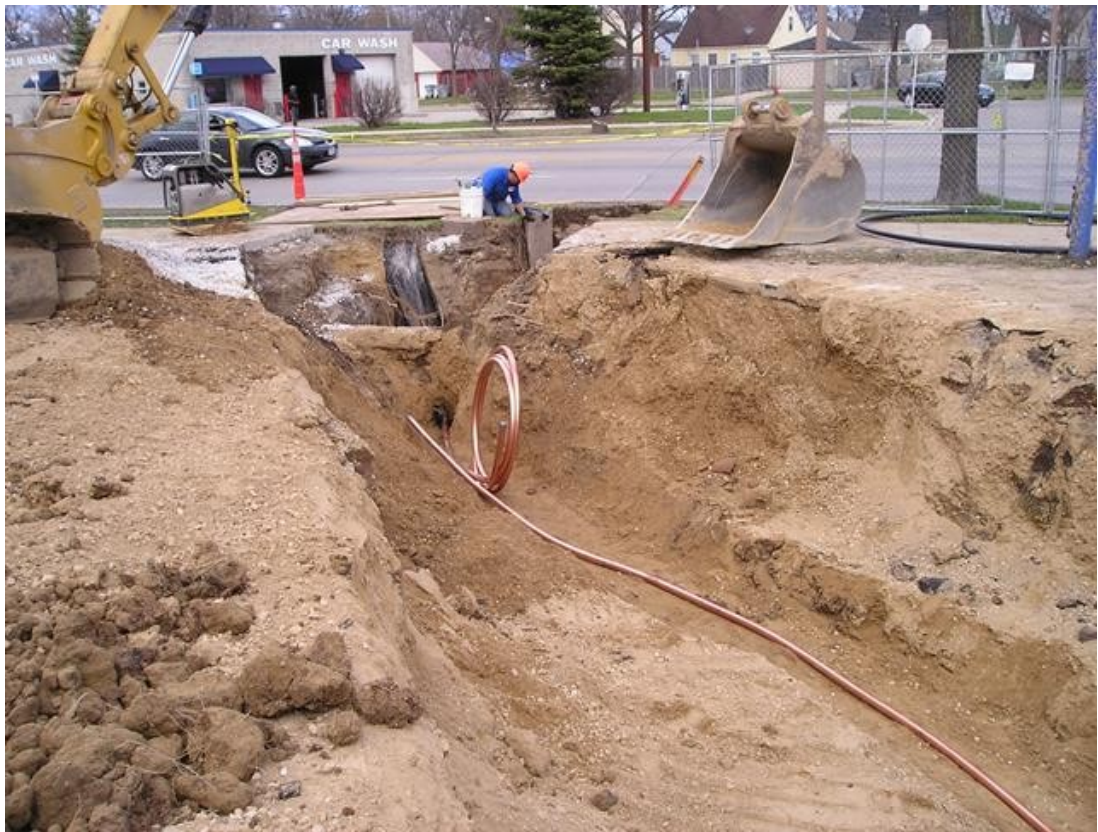
Below: Copper water lateral in the process of being connected to curb-stop.
