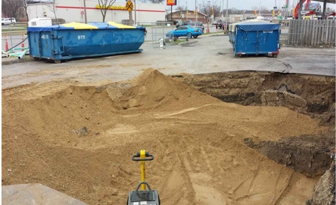
Above: Backfilling excavation and compacting in 1-foot lifts.
