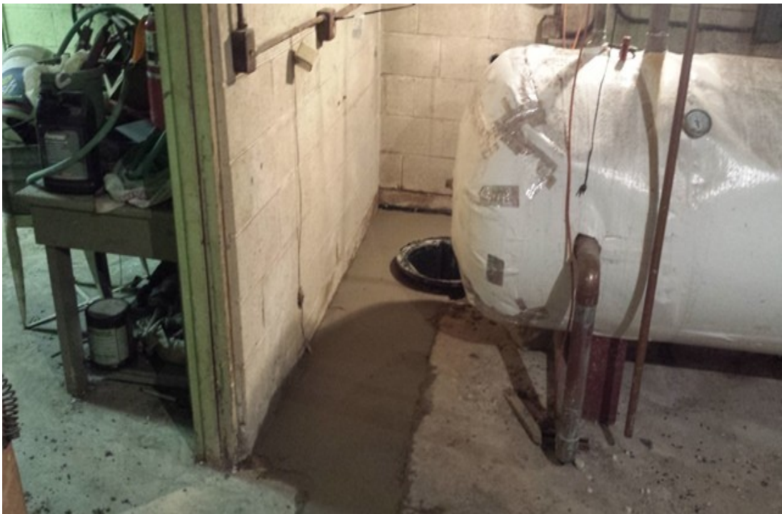
Below: Concrete restoration around new basement sump.
