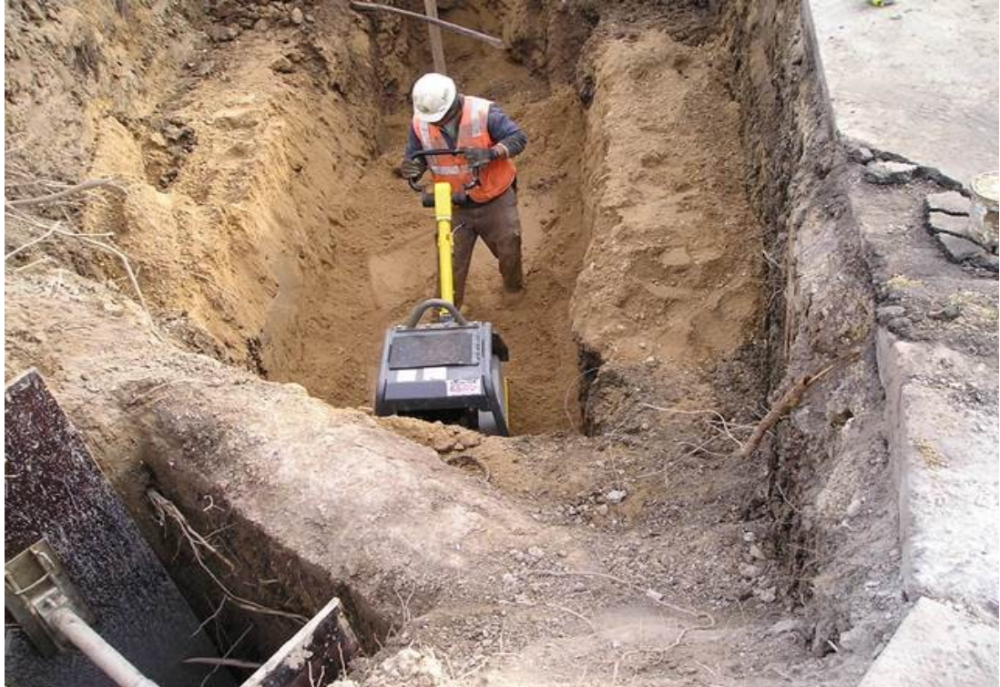
Below: Compacting of fill around and beneath the fiber optic cable and along the sanitary and water lateral trench near the sanitary main.
