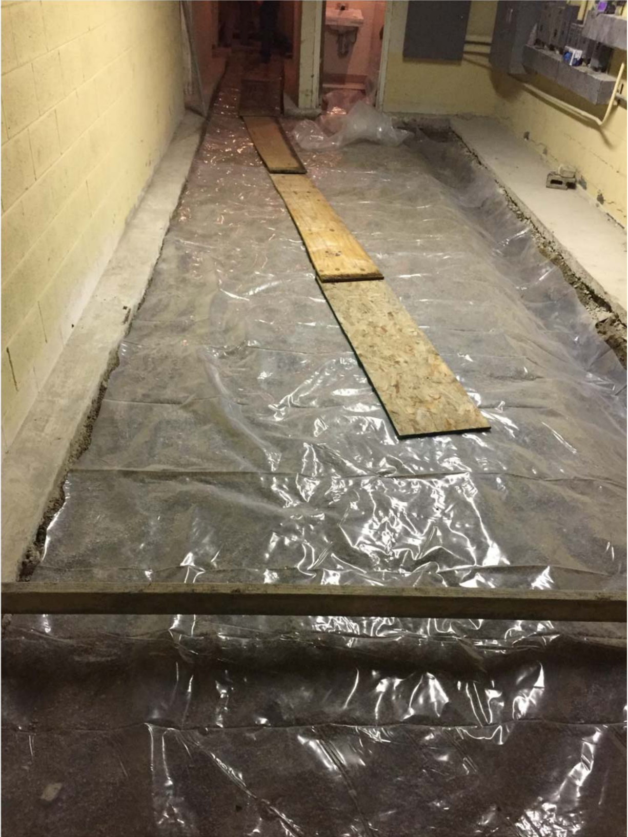
Vapor barrier and preparation for concrete slab replacement
