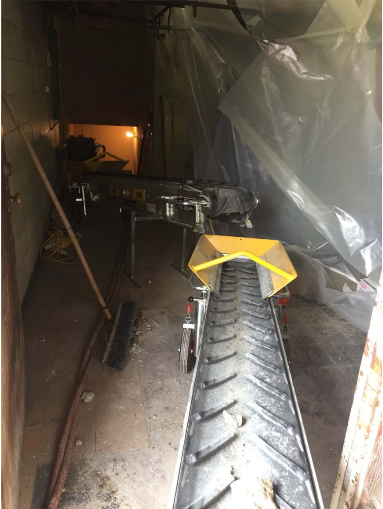
Conveyor moving material out the southeast building entrance. Facing west.
