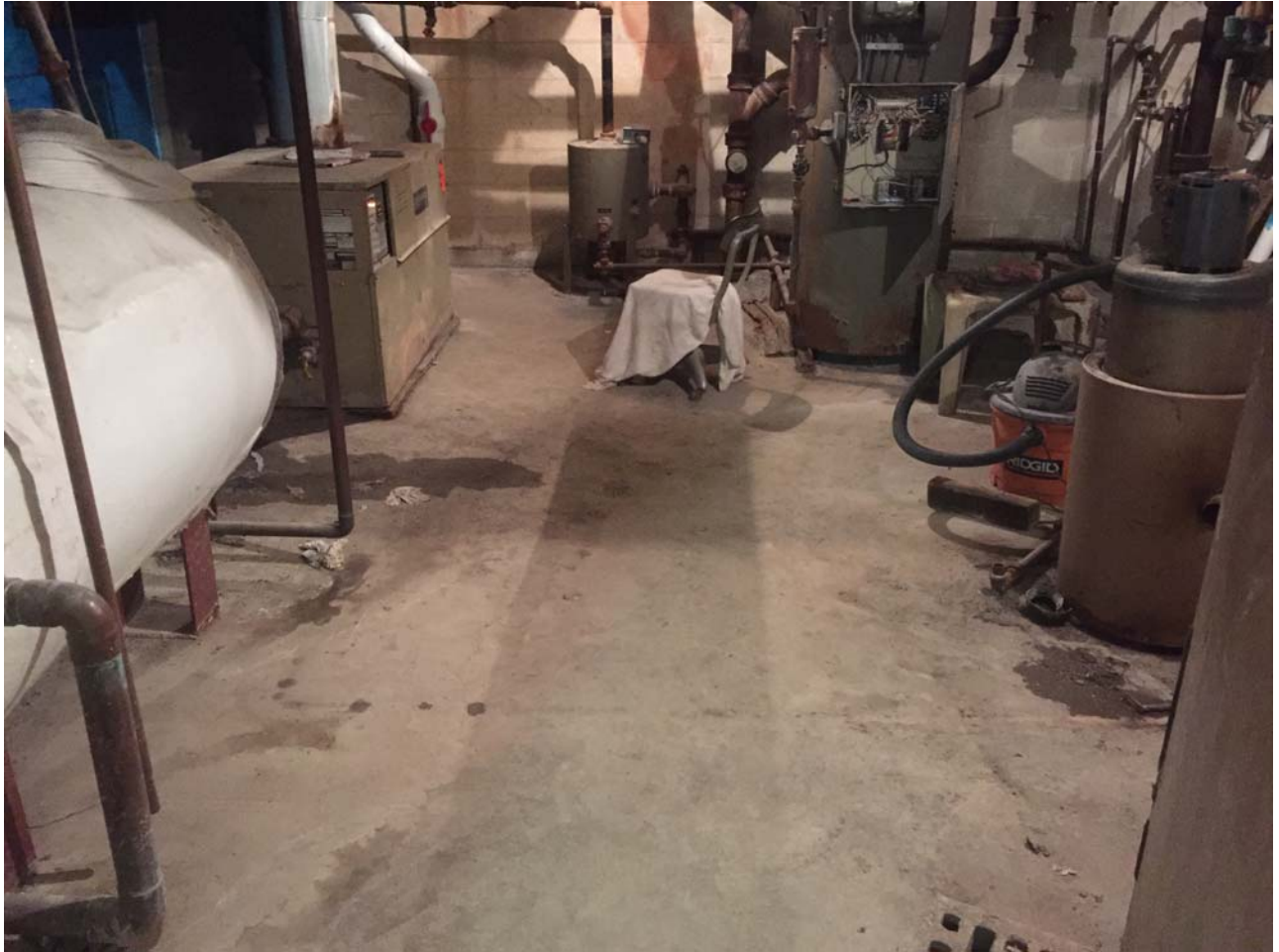
Basement mechanical room concrete floor slab
