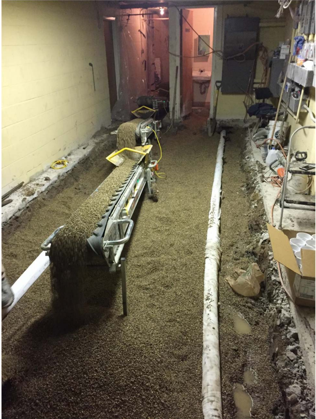
Horizontal vent pipes and pea gravel backfill in main storage room. Facing south.
