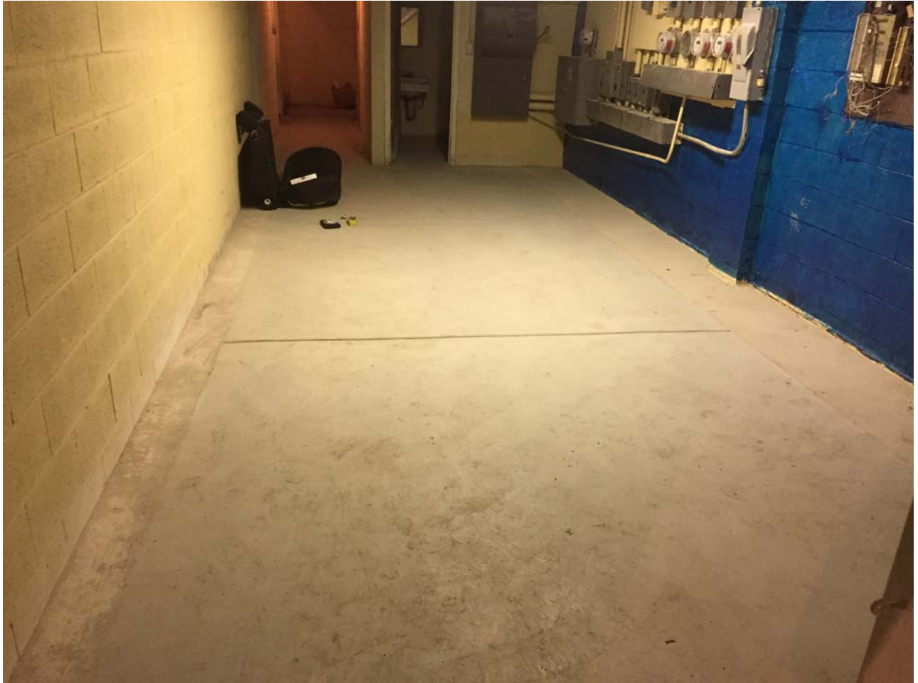
Basement concrete floor slab
