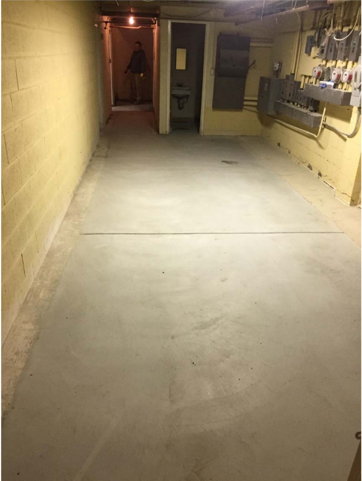
Excavation work completed.
