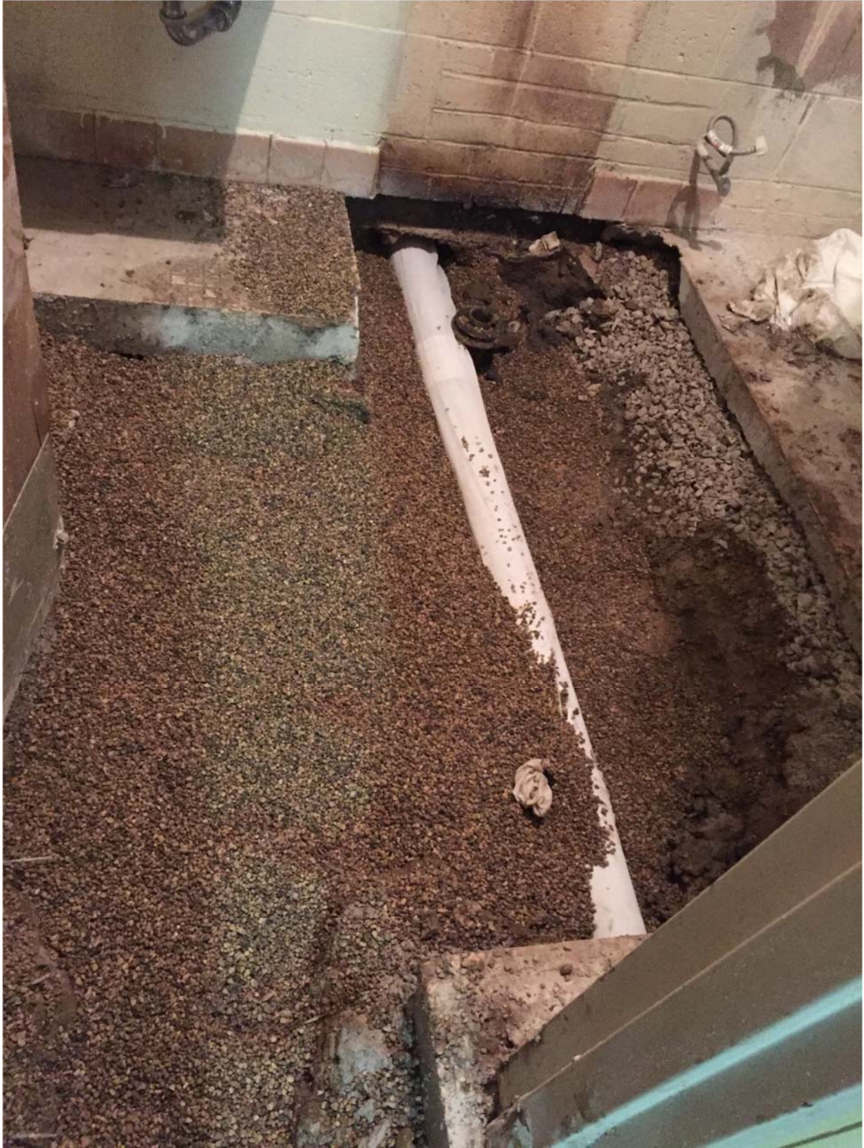
North restroom backfill and horizontal vent pipe.
