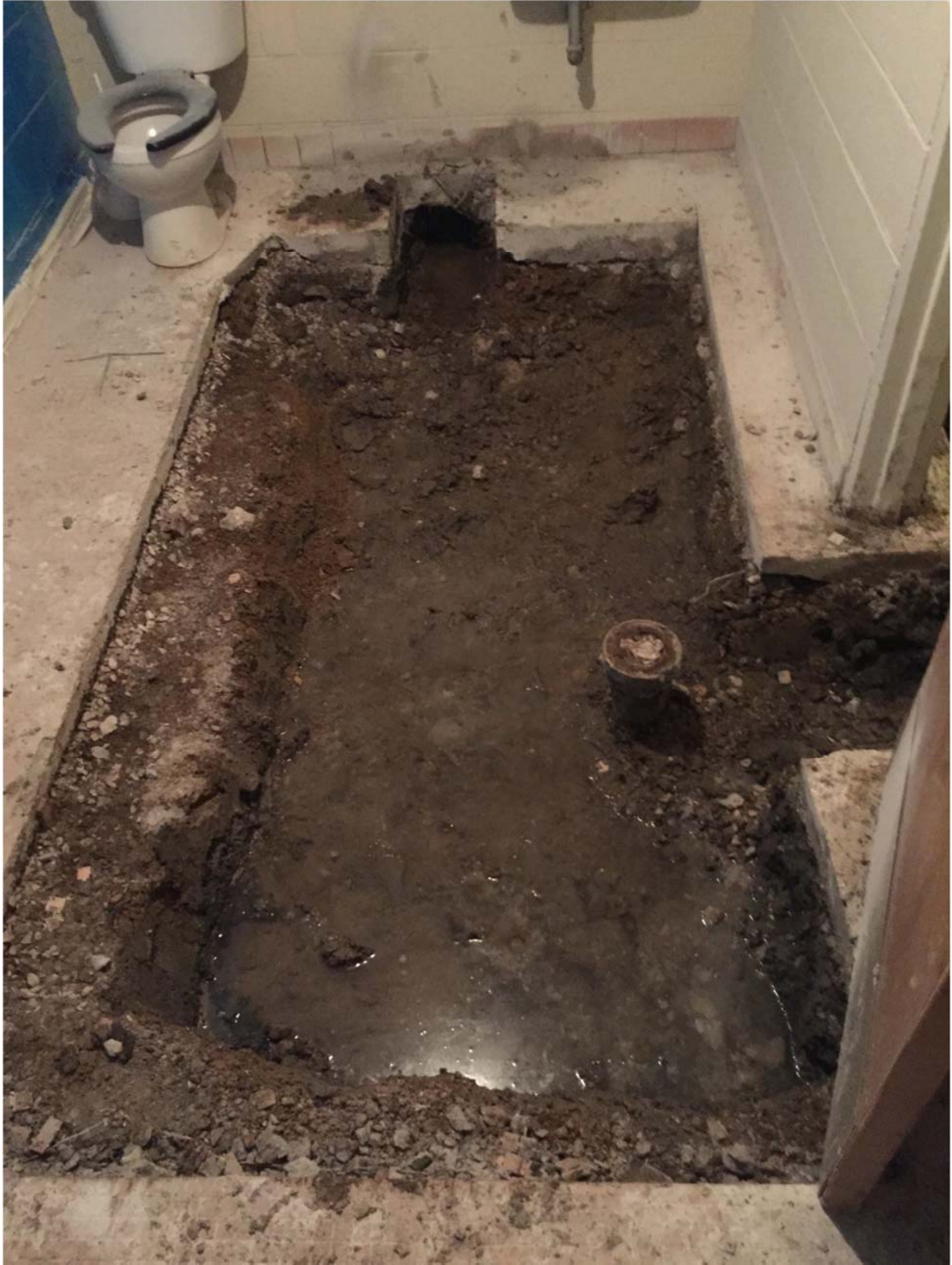
Excavation in south restroom.
