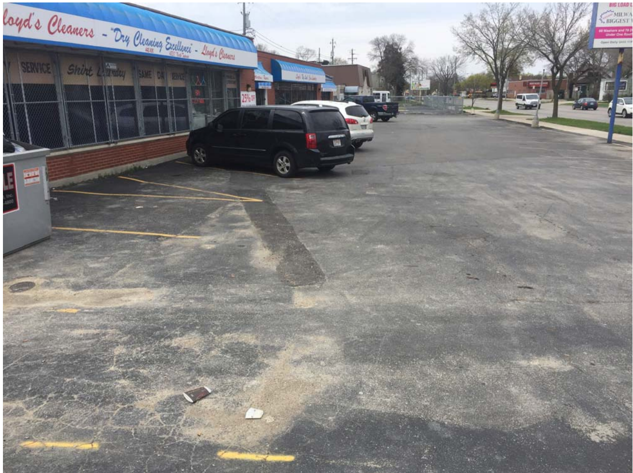
Overview of asphalt cap – facing north
