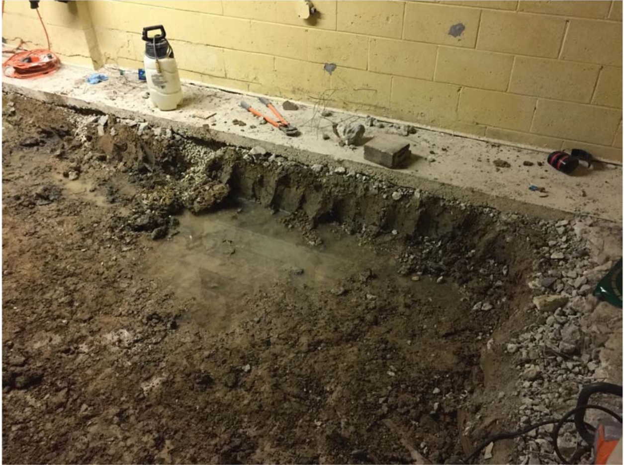
Soil excavation along west wall of storage room.
