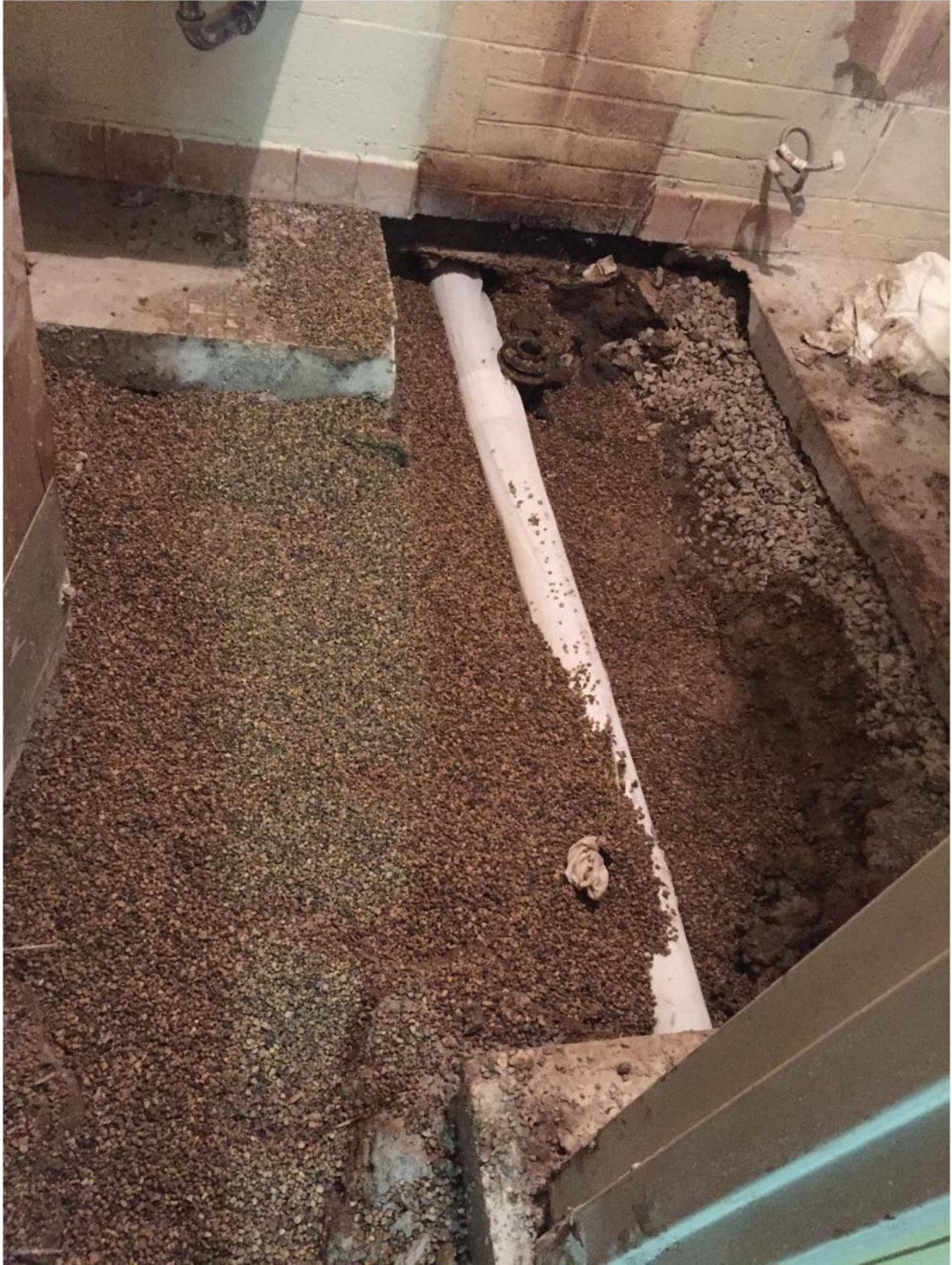
North restroom backfill and horizontal vent pipe.
