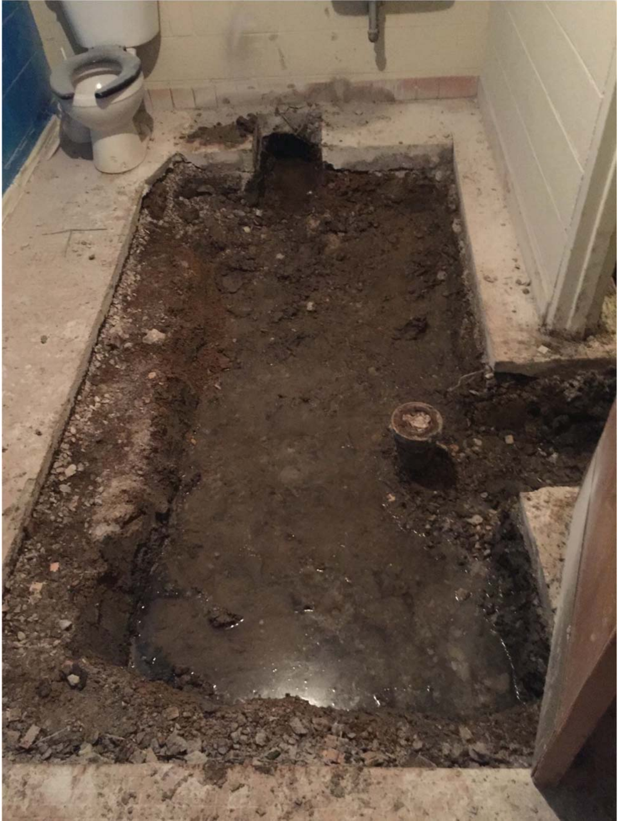
Excavation in south restroom.
