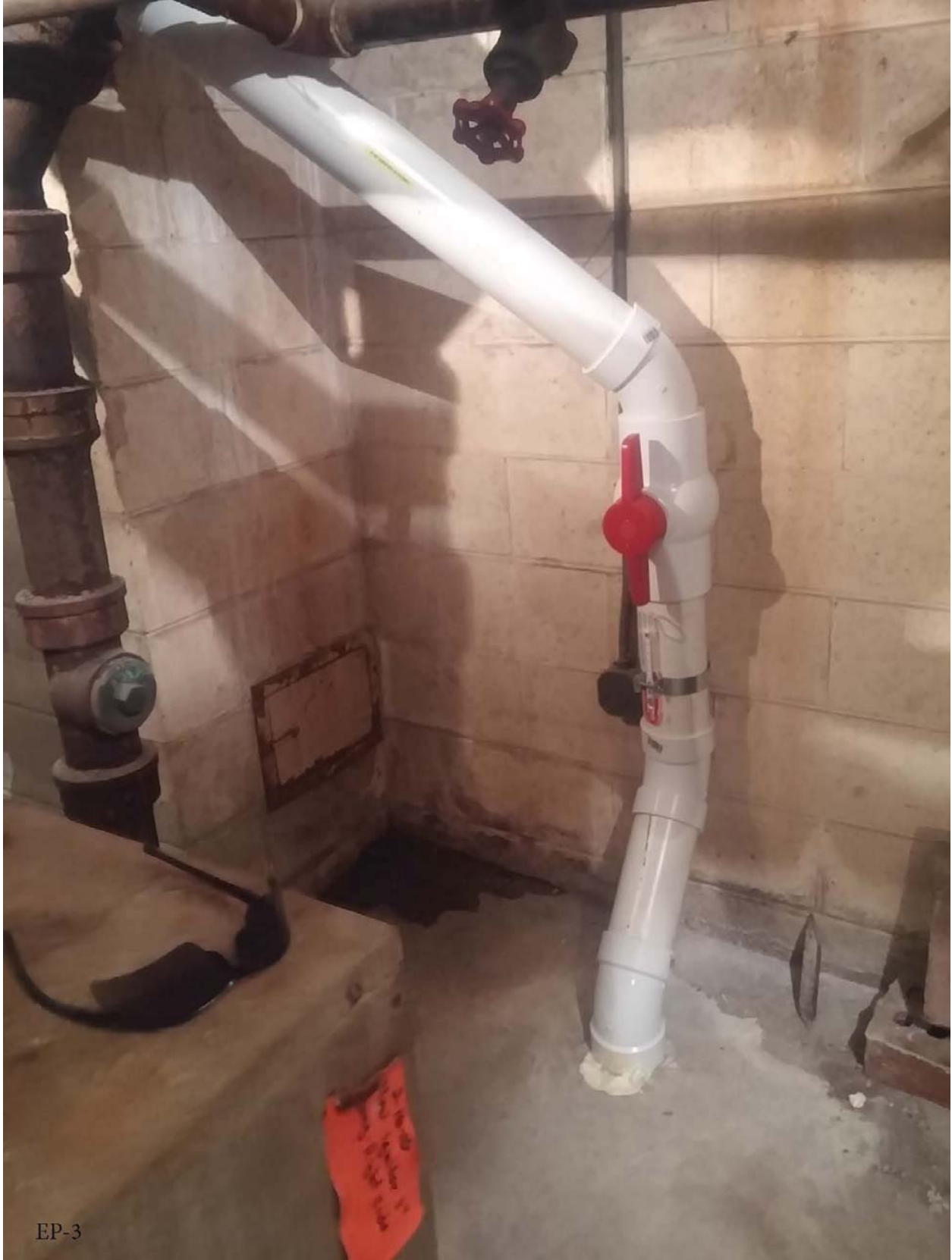
SSDS extraction point at north end of mechanical room.
