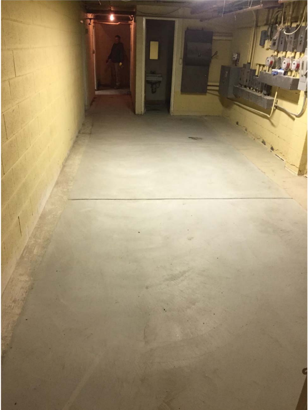
Excavation work completed.
