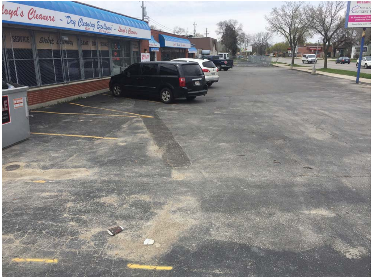
Overview of asphalt cap – facing north
