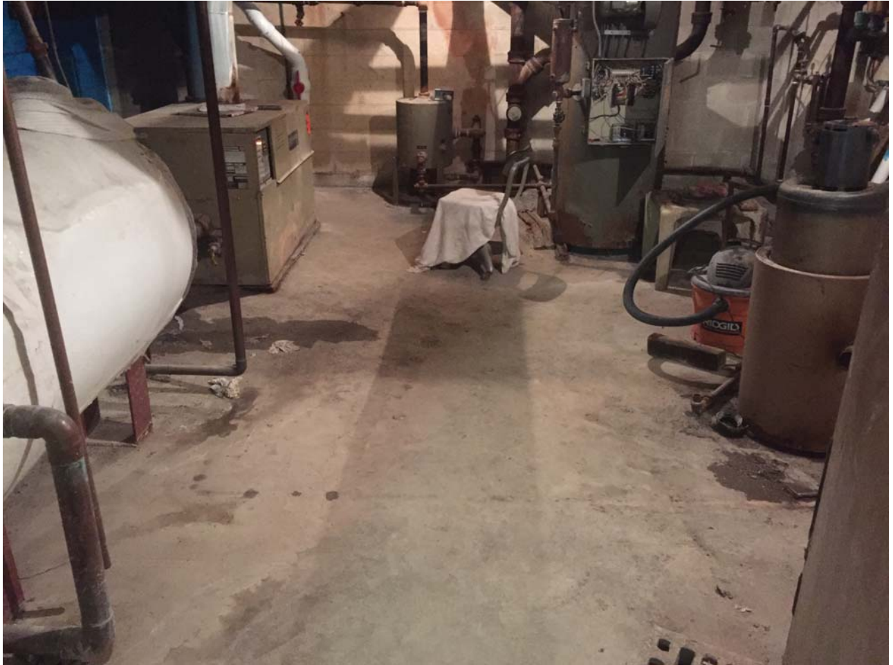
Basement mechanical room concrete floor slab
