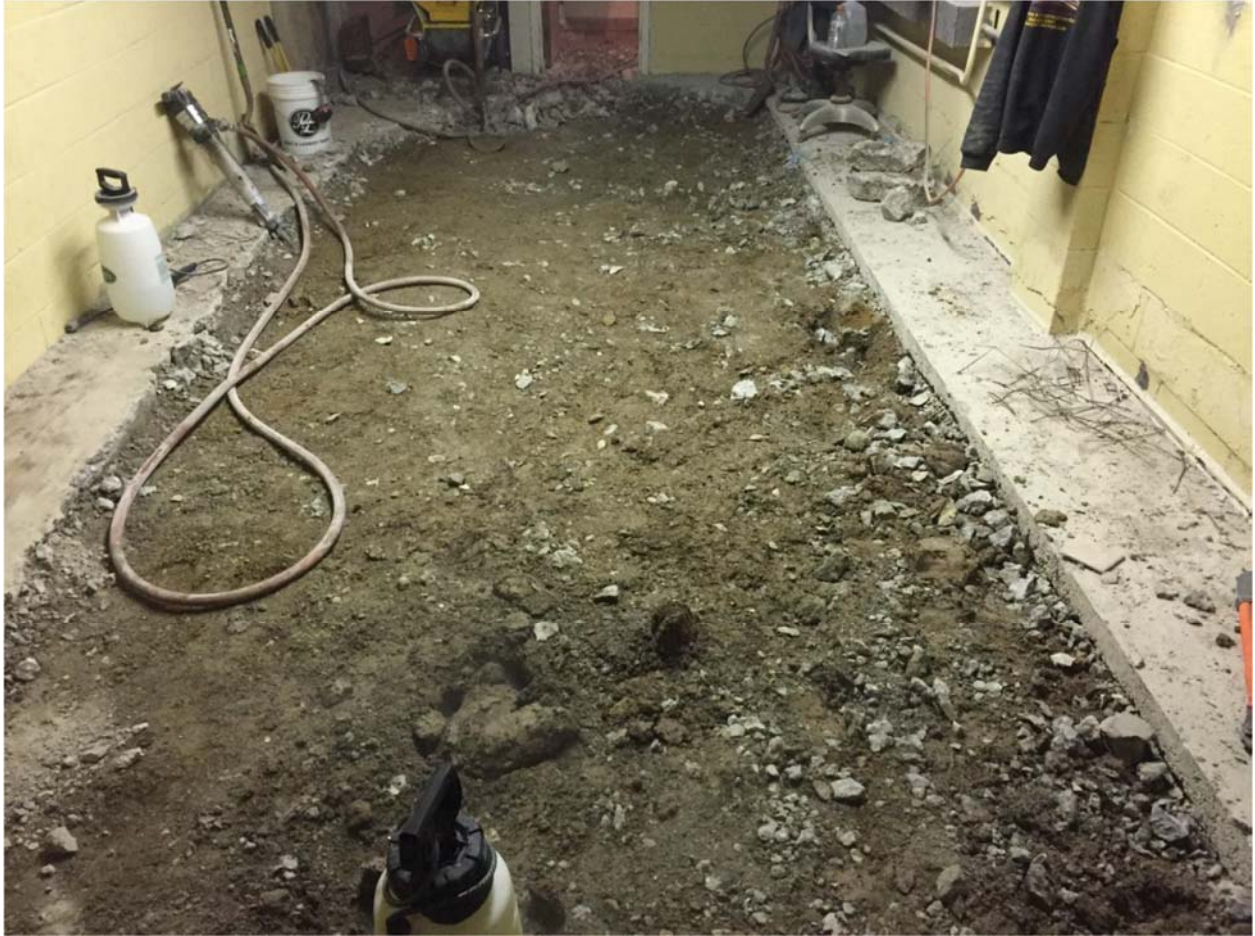
Main storage room with concrete slab removed. Facing south.
