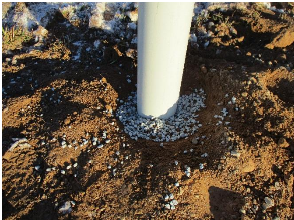
Photo #3 Photo of 6-inch casing seal that was set 1-foot into the bedrock at MW-9.
