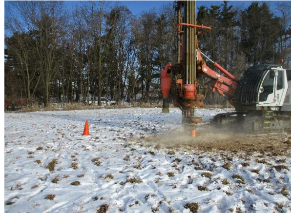
Photo #2 Photo looking north at installation of MW-9.
