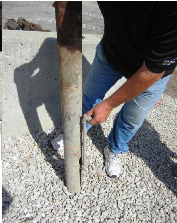
4) 4-inch pipe "sleeved" over 1-inch line valve.
