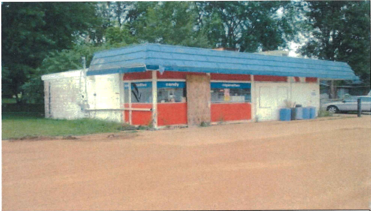
Photograph of the Northwest corner of the subject site, viewing southeast towards the structure.
