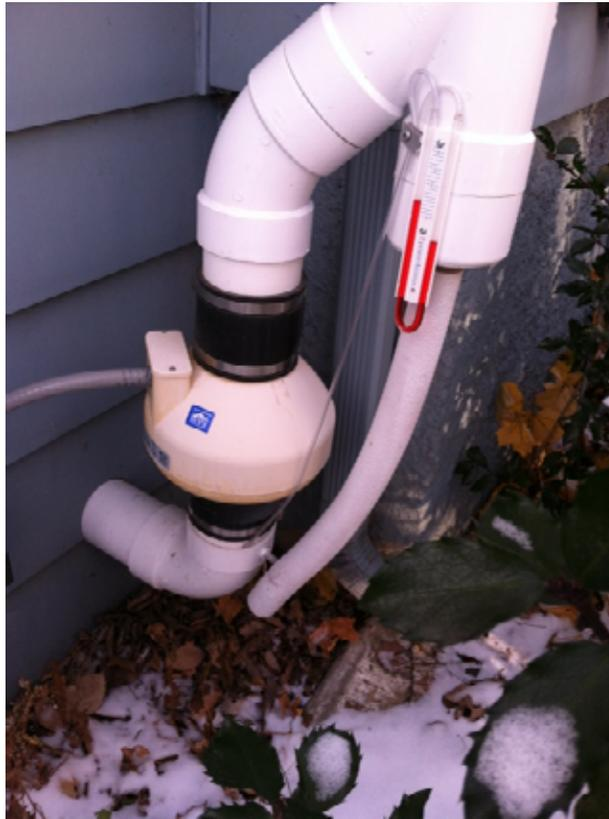
Crawlspace SSDS manometer, operating level 0.9 in wc
