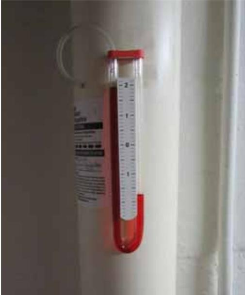
Basement SSDS manometer, operating level 3.6 in wc
