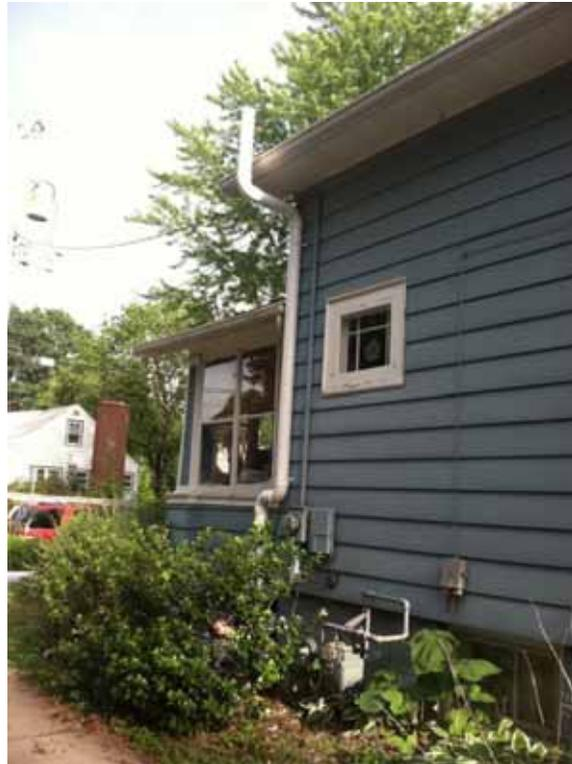
Crawlspace SSDS fan and discharge piping
