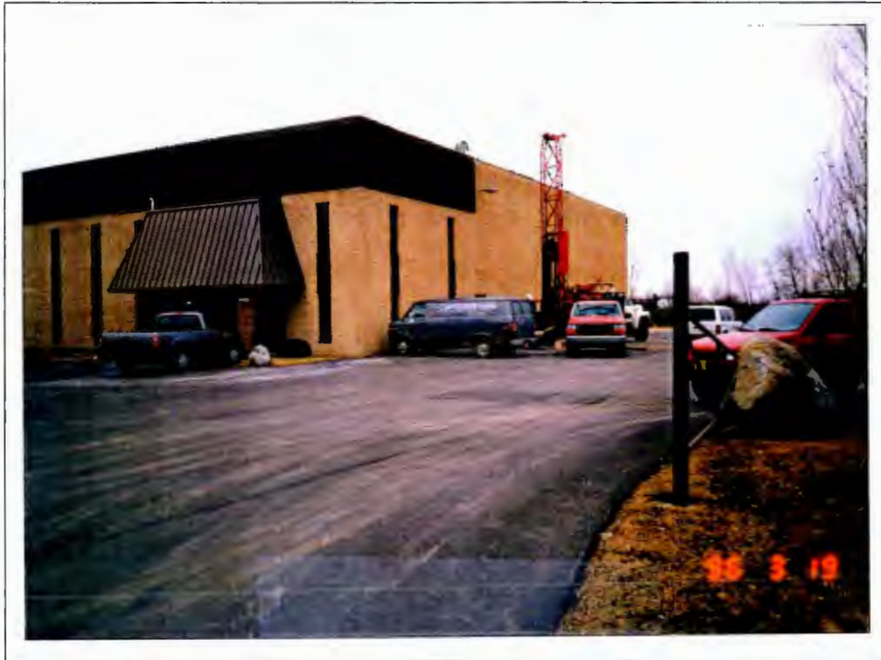
Photo taken facing northwest toward southeast building corner.
