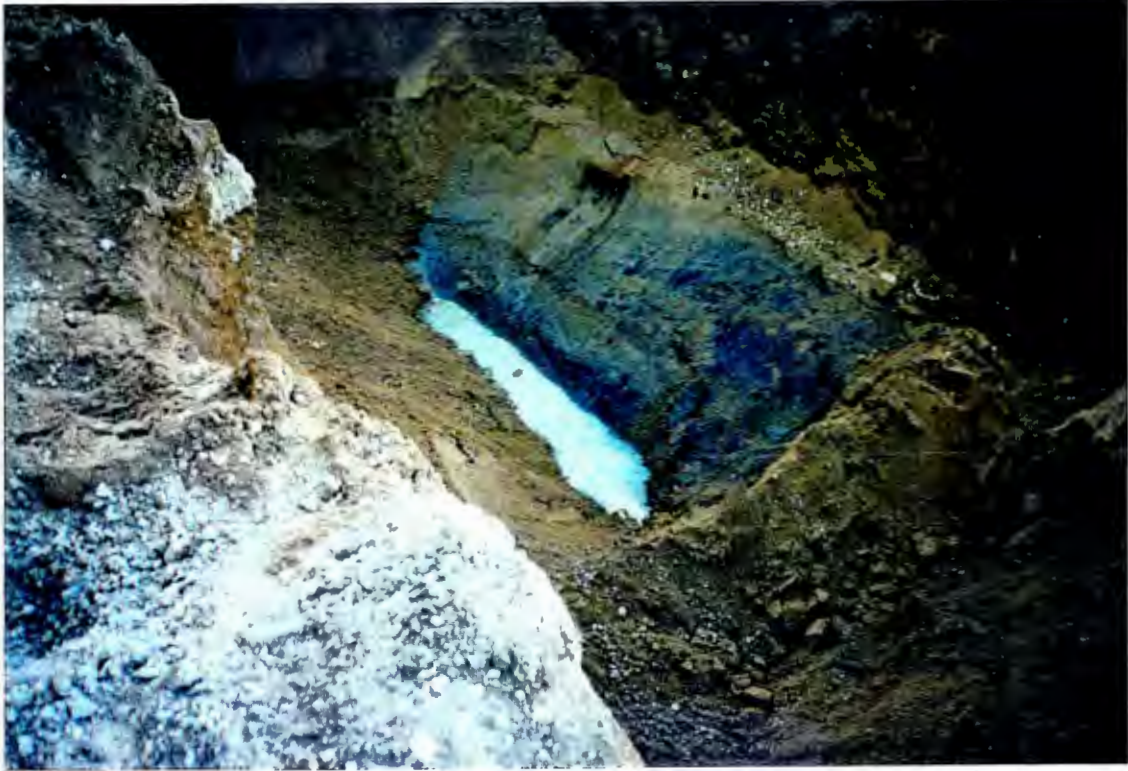
Photo shows perched water at bottom of northern tank.
