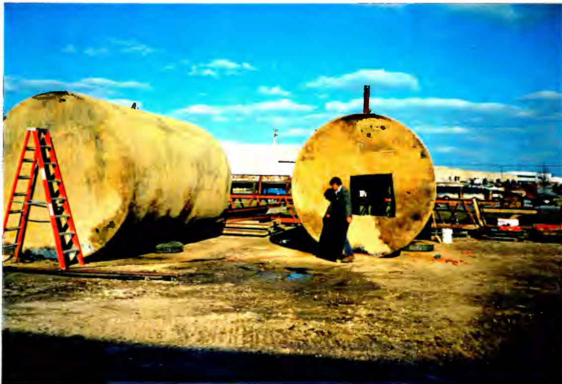
Cleaning of one 10,000 gallon tank by Northern Petro Services, Inc.
