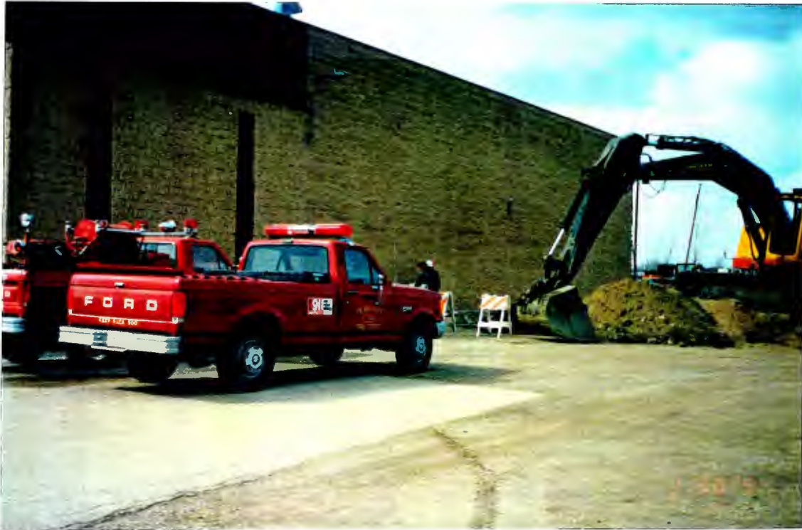
UST removal activities in 1994.
