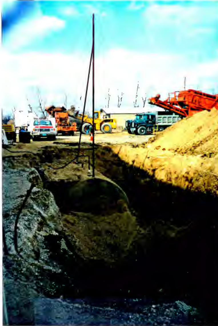
Photo shows venting of northern tank prior to removal.
