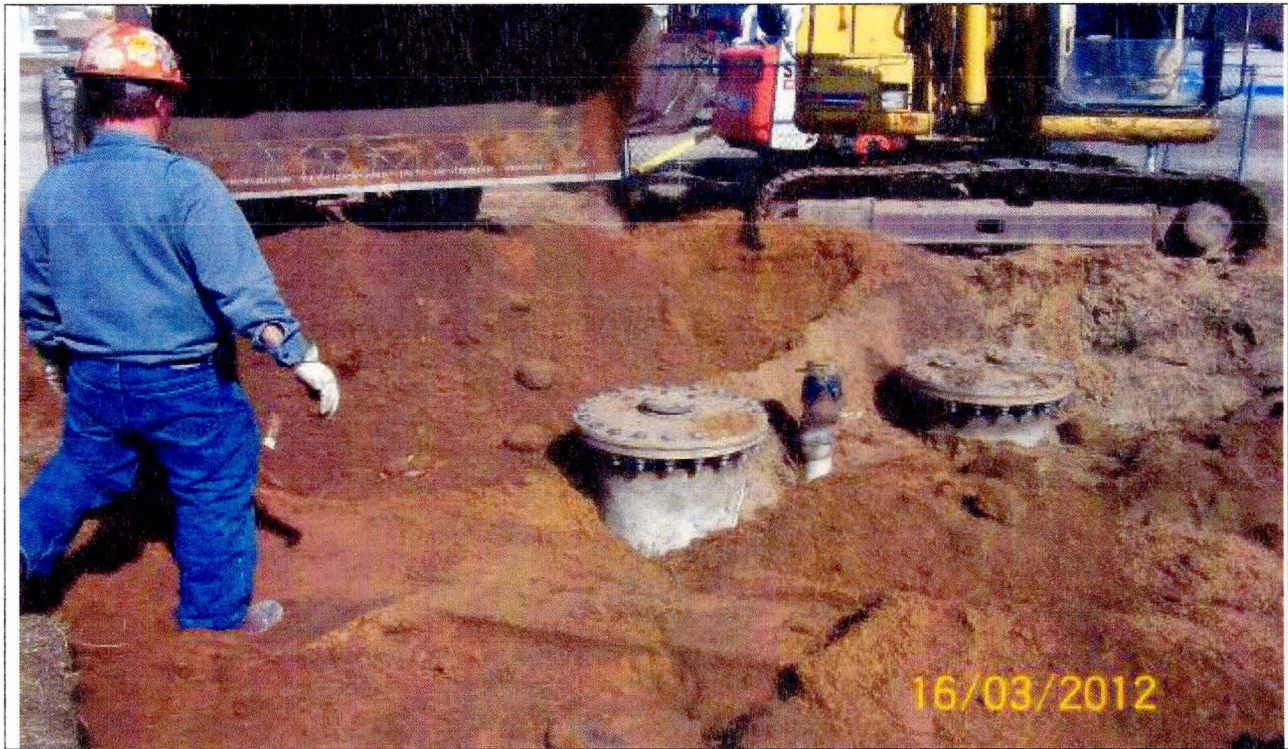
Picture 7: Clean fill replacing removed contaminated soils.
