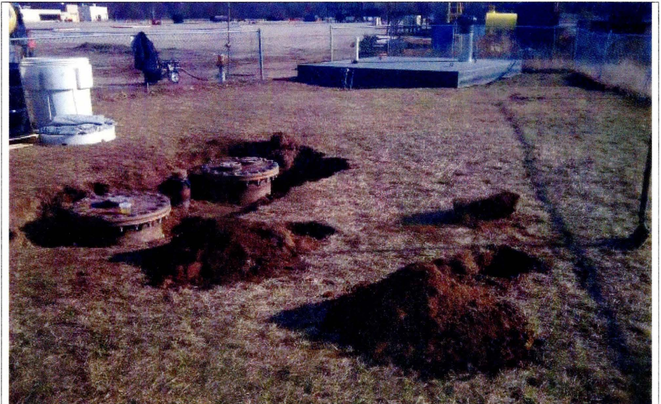
Picture 2: Initial removal of the contaminated soils.
