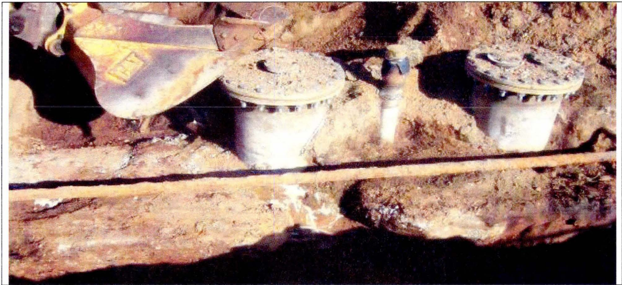
Picture 5: Removing contaminated soils.
