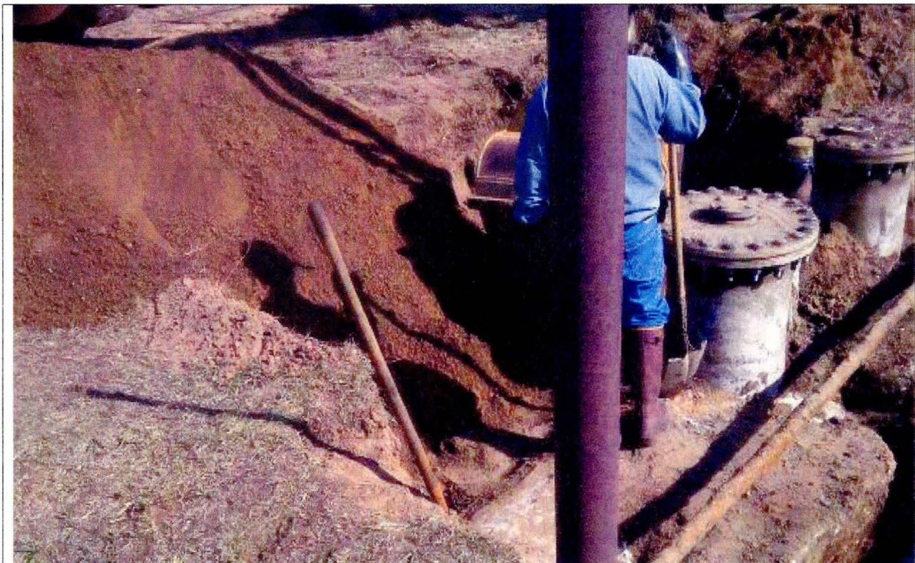
Picture 6: Clean fill added to the spill area.
