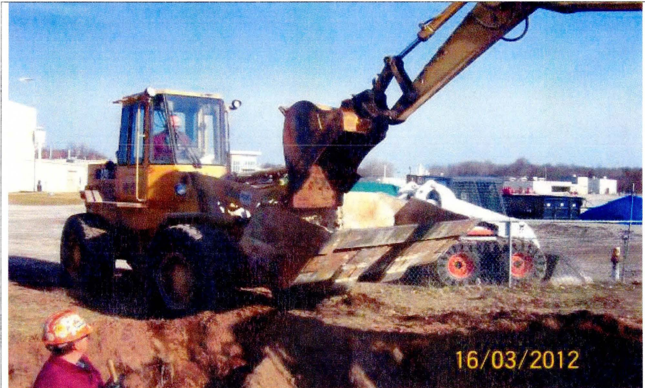
Picture 3: Veolia removing the contaminated soils to the Roll-off.
