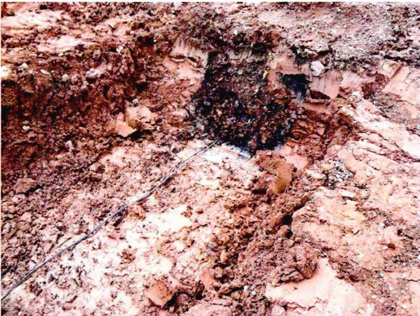
Photo 6: Contaminated soil following cathodic line near northeastern mixer excavation. April 9, 2012.
