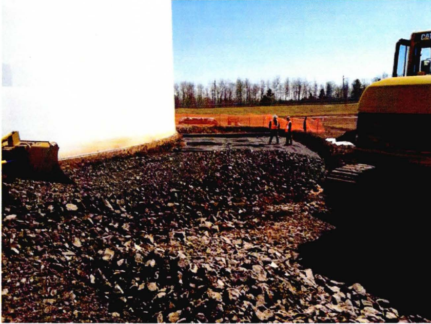
Photo 1: Ring road construction near western manway. April 3, 2012.
