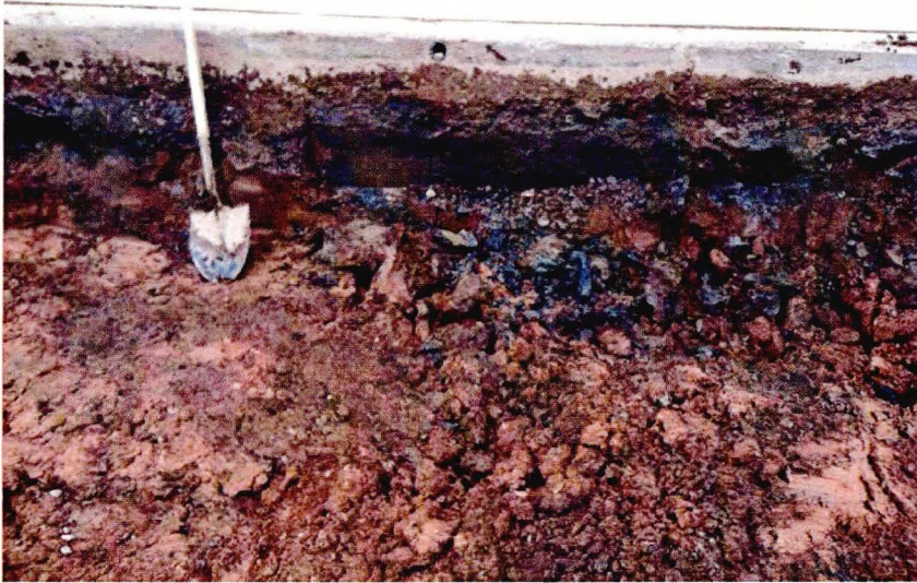
Photo 5: Contaminated soil left in place near northeastern mixer excavation. April 9, 2012.
