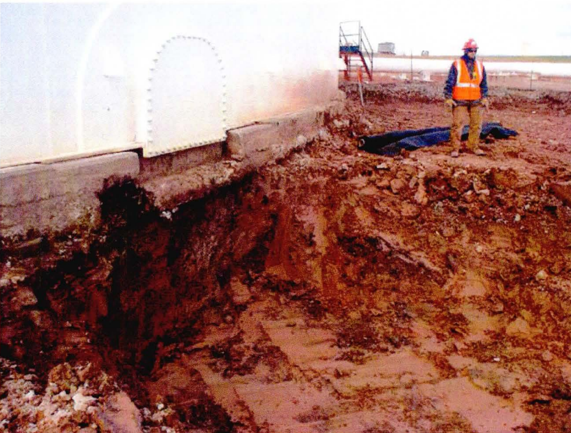
Photo 4: Final northern D-door excavation. April 9, 2012.
