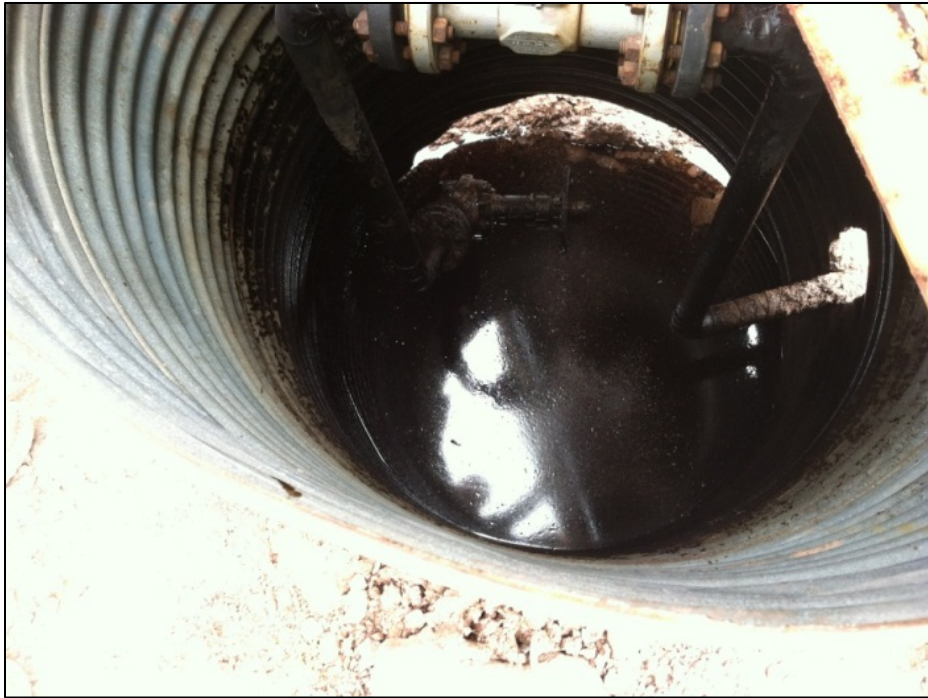
Photo 3: Whistle containing free product. The whistle was removed during hydrotest excavation activities.
