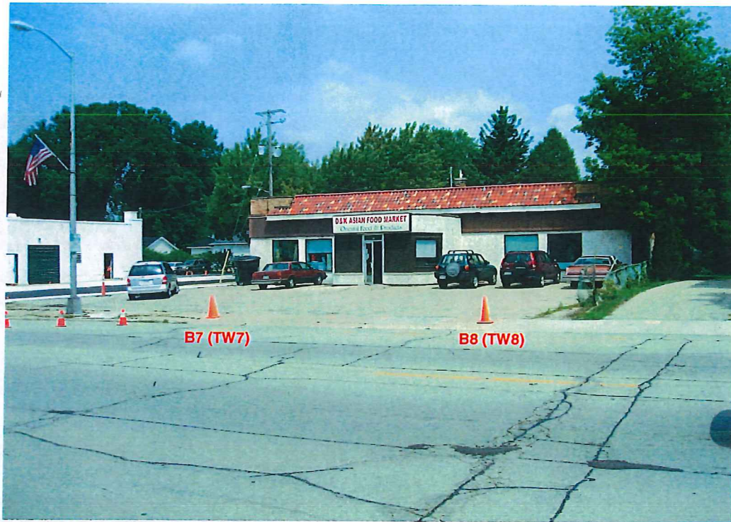
Photo and Plan View of Site, Showing Boring Locations D & K Asian Food Market, 122 W. Wisconsin Ave.
