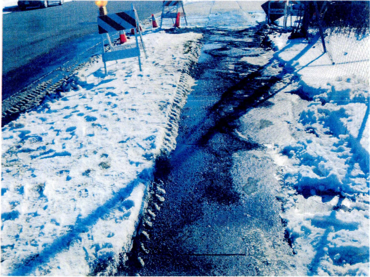
Area with Oil Dry applied
