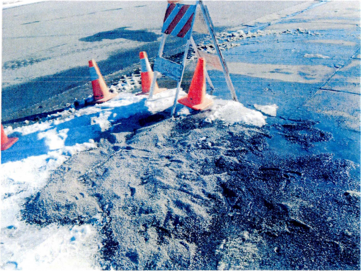
Area with Oil Dry applied
