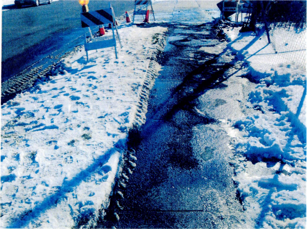
Area of Product with Oil Dry Applied
