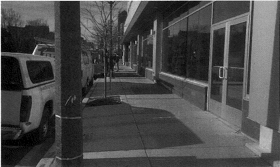
Photo 22: Exterior of south side of building with concrete sidewalks and W. Wells Street to the left (view to west; December 2, 2014).
