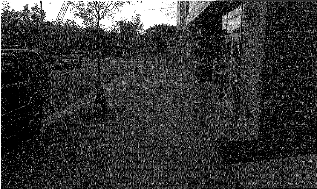
Photo 21: Exterior of east side of building with concrete sidewalks and N. 14th Street to the left (view to south; September 29, 2014).
