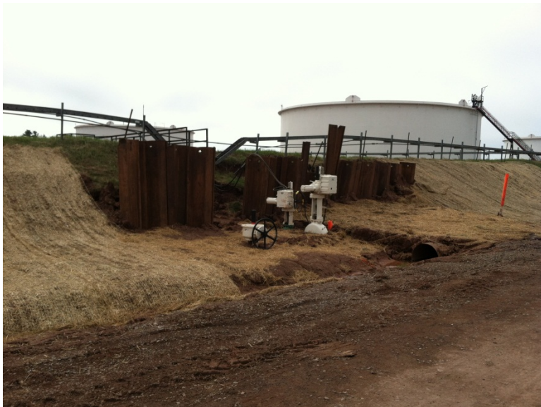
Photo 3: Backfilled valve excavation. (5/3/2012)
