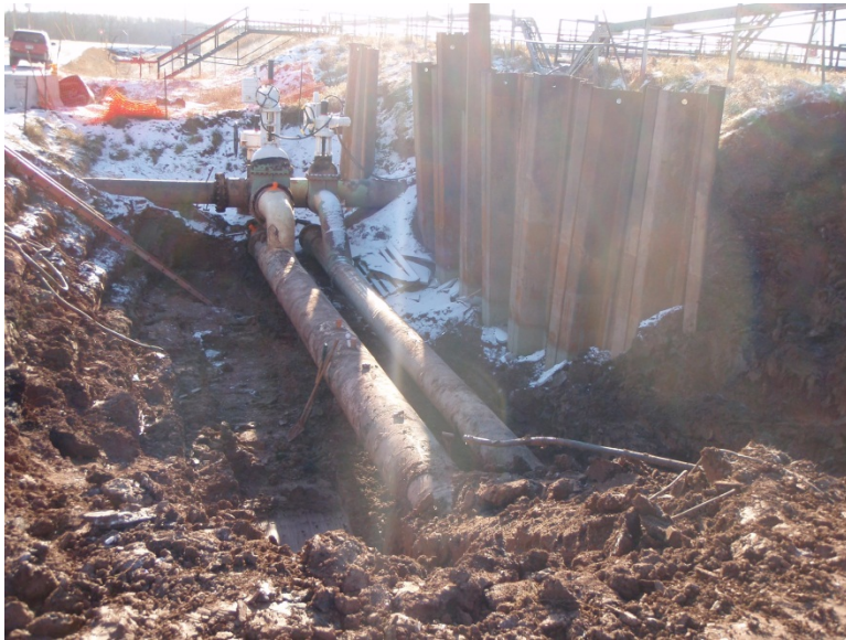
Photo 2: Expanded excavation required for valve repair work. (12/6/2011)
