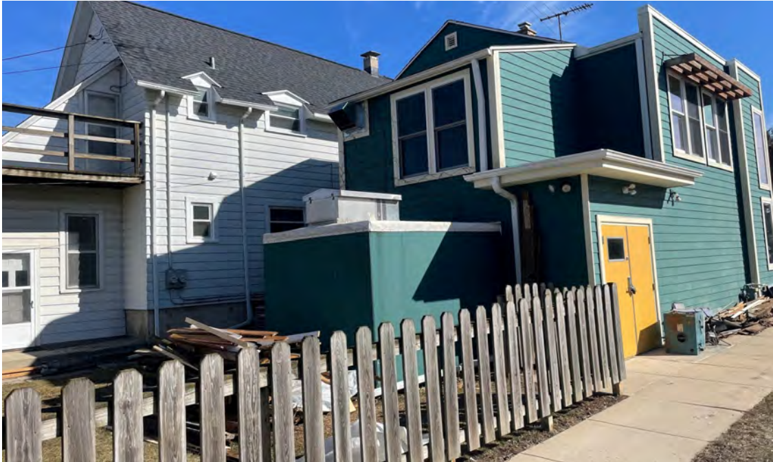
Photo 3: View of west side of 1229 12th Avenue building. View to northeast. 3/8/2023.
