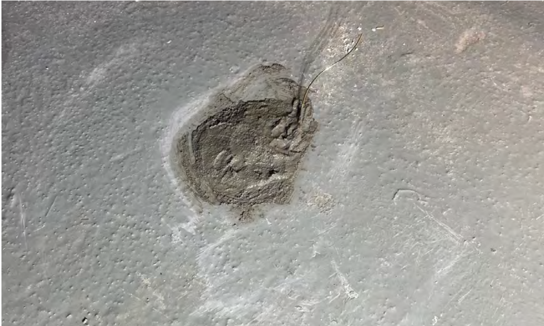
Photo 3: Sub-slab sample point SSV-01 in the basement of the 1229 12th Avenue building following installation of the temporary cement cap. 3/22/2023
