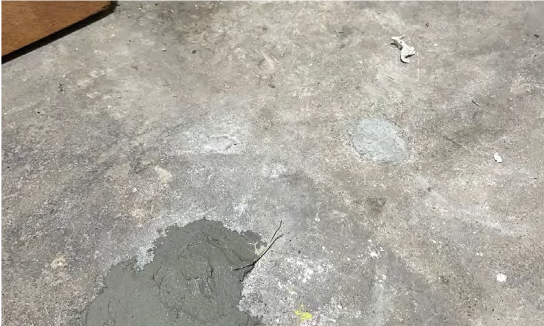
Photo 5: Sub-slab sample point SSV-02 in the 1233 12th Avenue building following installation of the temporary cement cap. Previous SS-2 sample location visible. 3/22/2023.
