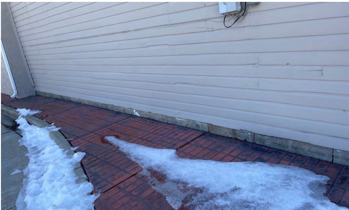
Photo 6: View of northwest exterior of 1233 12th Avenue building. View to southeast. 3/8/2023.
