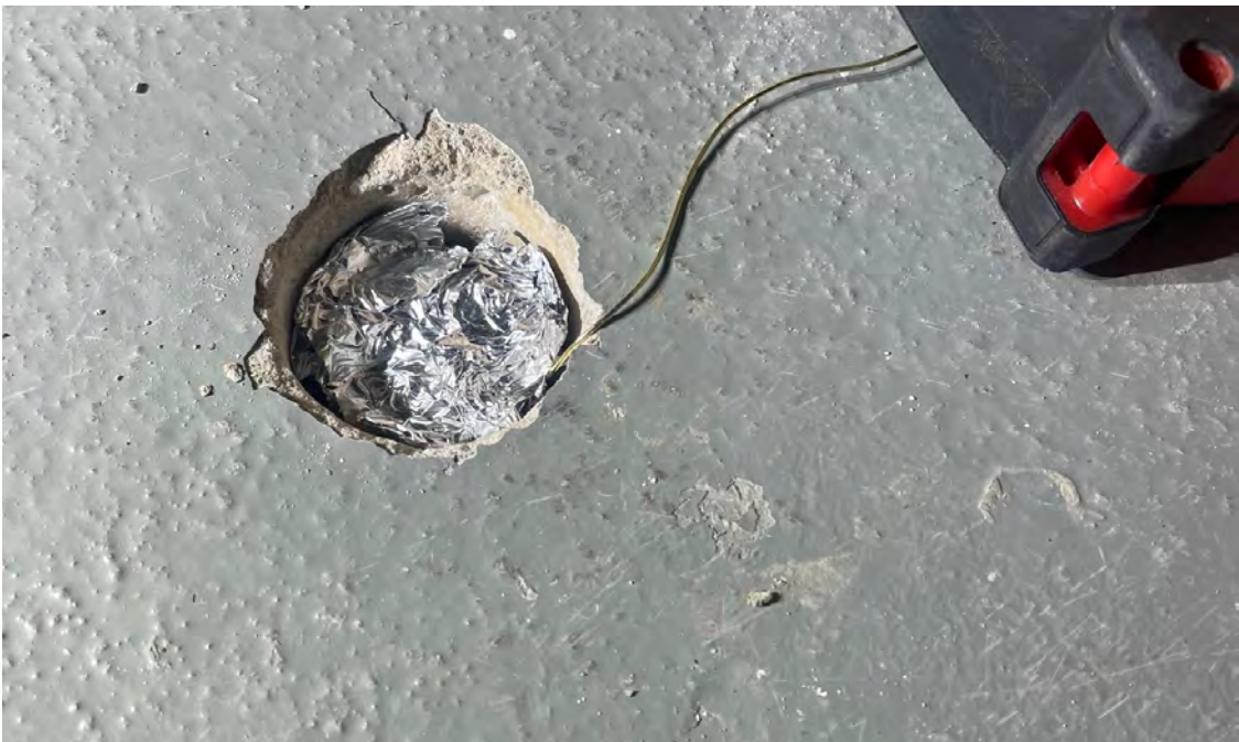
Photo 2: Sub-slab sample point SSV-01 in the basement of the 1229 12th Avenue building following installation of the passive sampler and capping with aluminum foil plug. 3/22/2023
