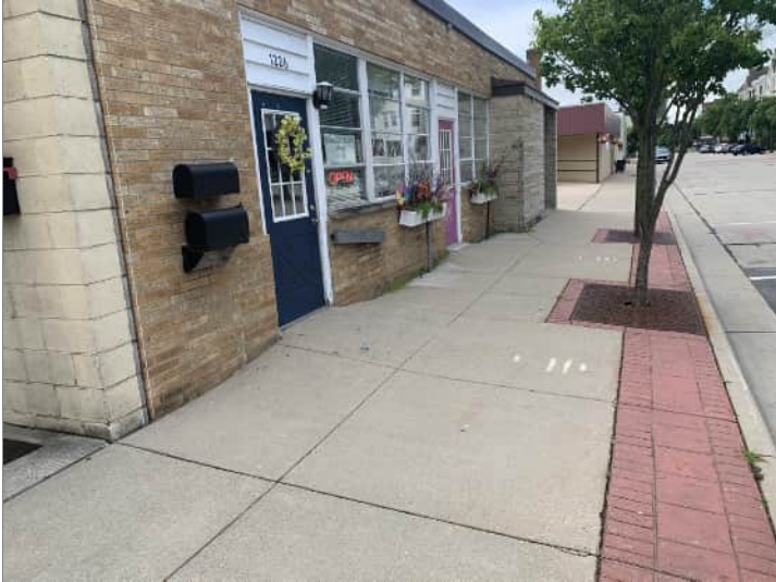
Title: West side of building (facing S/SE)
