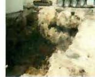
CONTAMINATED SOIL EXCAVATIONS
