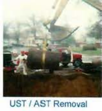
UST / AST Removal
