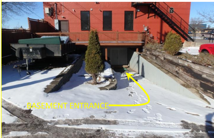
South side of building showing basement entrance.
