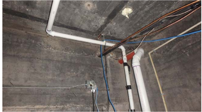
Ventilation piping for Radon System
