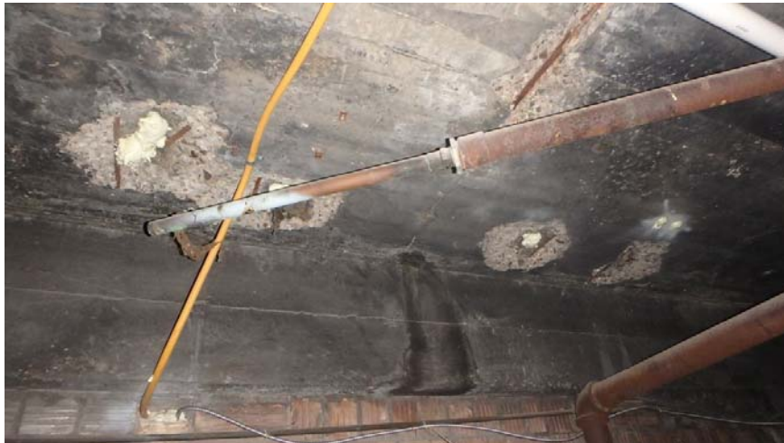
Sealed holes in ceiling
