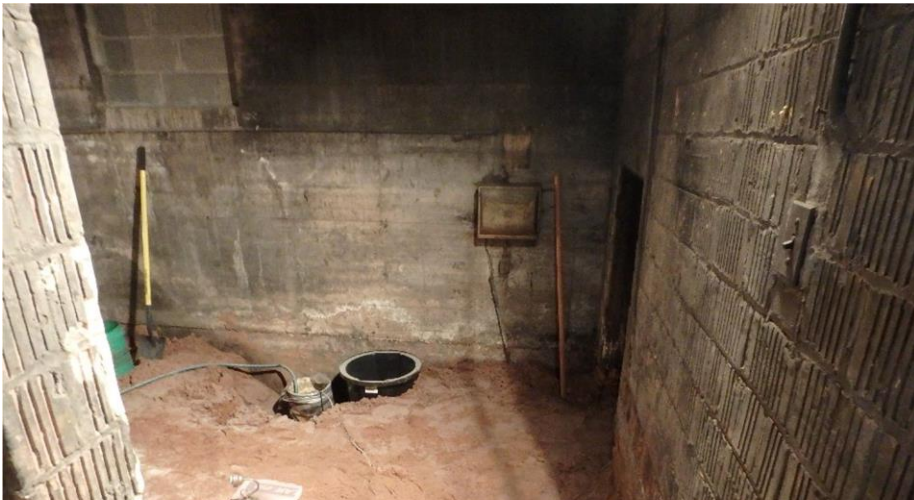
View of sump after installation.
