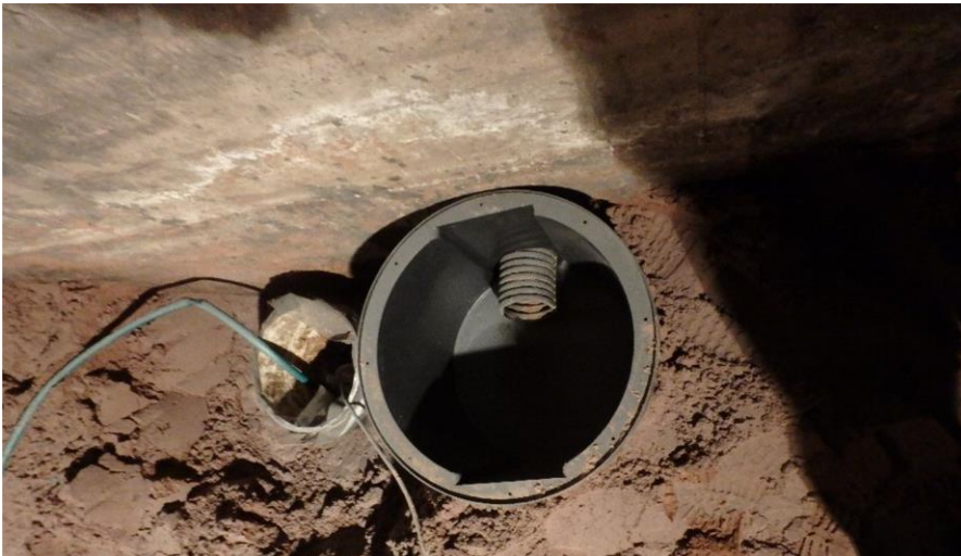
Close up view of newly-installed sump.
