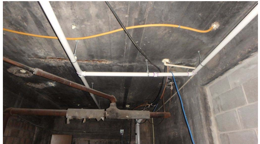
Ventilation piping for Radon System
