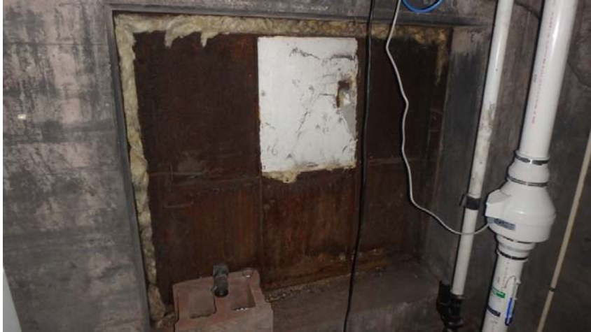
Sealed entryway behind Radon System
