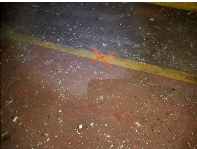
Photo 23) Typical Floor Stripe with Lead-Based Paint
