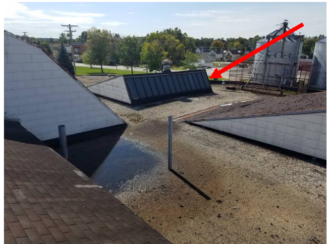
Photo 5) Window Glazing – Bldg 3 Skylights
