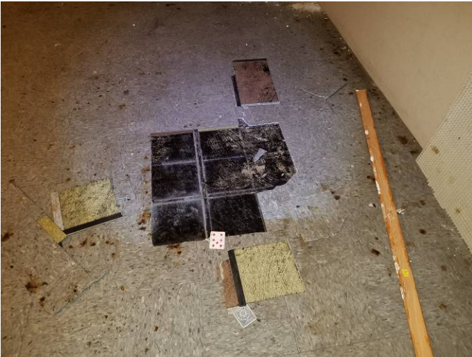
Photo 13) 9" Tan Floor Tile & Black Adhesive - Bldg 15 Mezzanine
