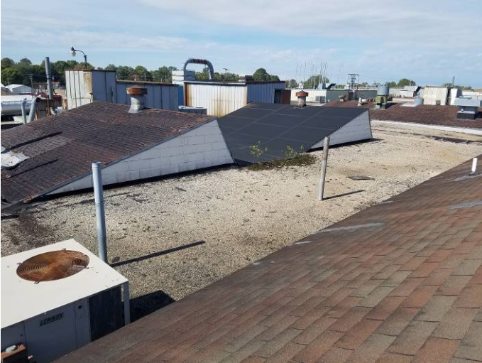
Photo 1) Transite Siding – Bldg 3 Roof
