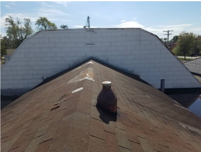
Photo 2) Transite Siding – Building 2 Roof
