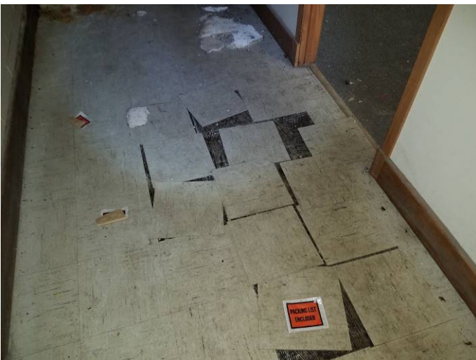
Photo 15) 12" Tan Floor Tile & Black Adhesive - Bldg 1 Offices
