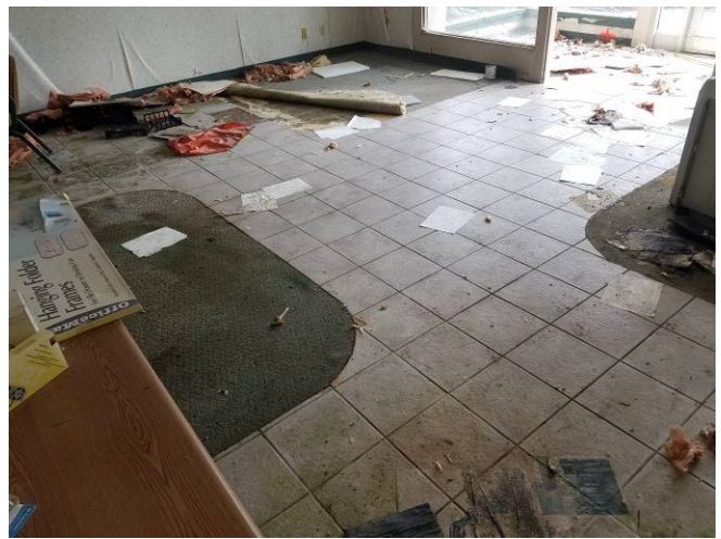
Photo 18) Black Flooring Adhesive - Bldg 1 Lobby
