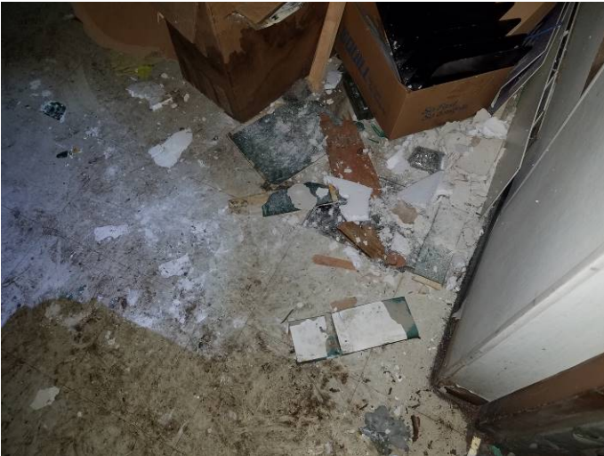
Photo 14) 9" Green Floor Tile & Black Adhesive - Bldg 11 Offices
