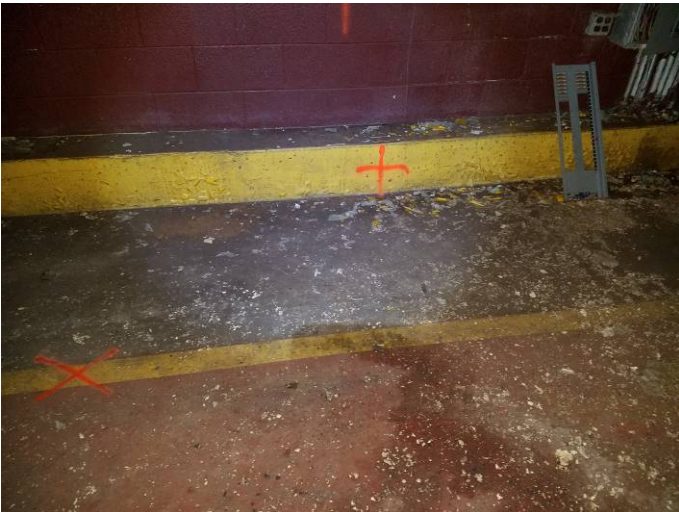
Photo 22) Typical Curb with Lead-Based Paint
