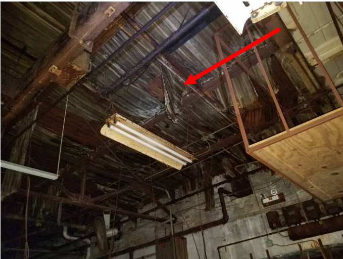
Photo 8) Brown Roofing Paper – Bldg 3
