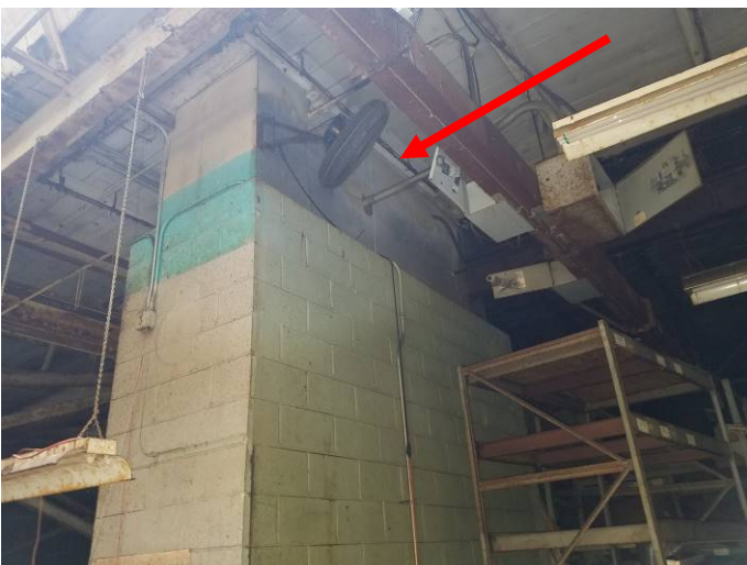
Photo 9) Transite Paneling – Bldg 3
