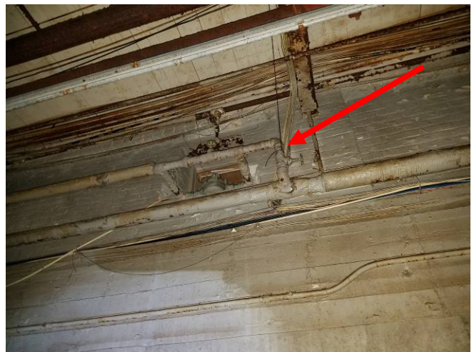
Photo 6) White Pipe Insulation – Bldg 2 (west wall – upper)
