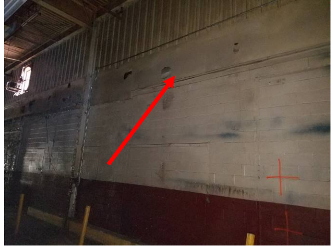
Photo 10) Transite Paneling – Bldg 17
