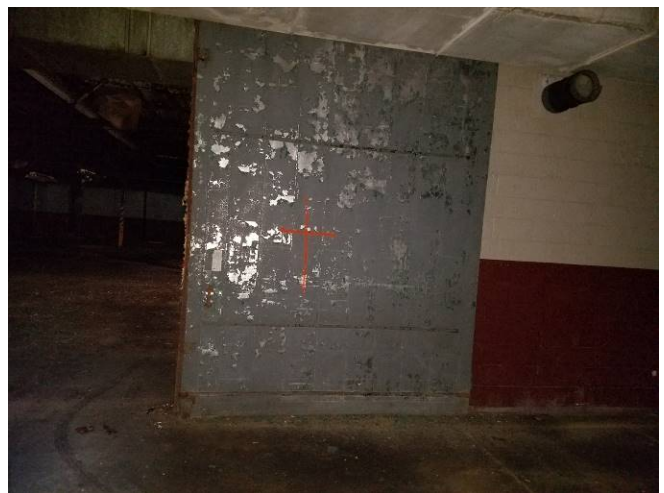
Photo 12) Typical Fire Door
