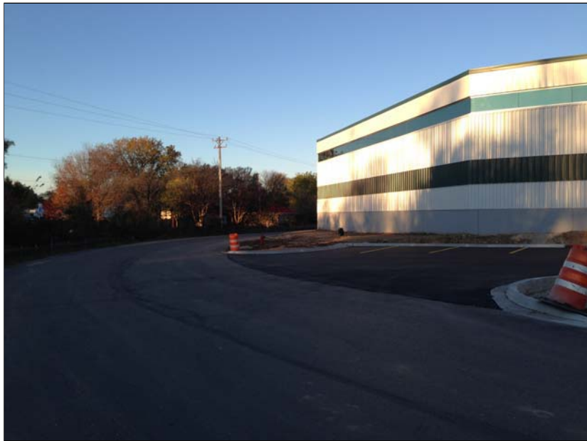
Photo 2: Southeast corner of building addition and paved areas, looking southwest
