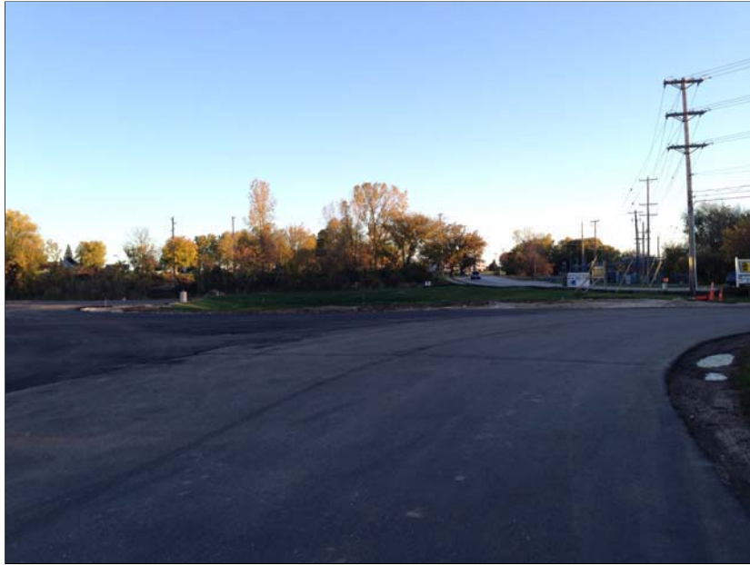
Photo 5: Driveway, parking areas, and stormwater management pond, looking north
