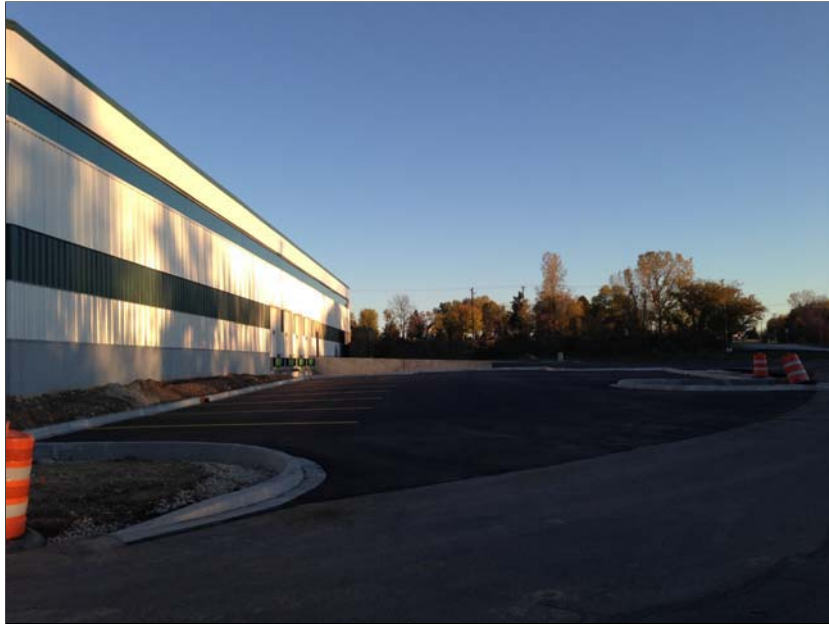
Photo 3: East side of building addition and paved parking areas, looking north
