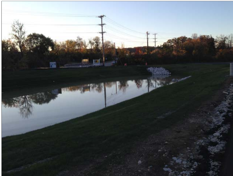
Photo 6: Stormwater management pond, looking southeast
