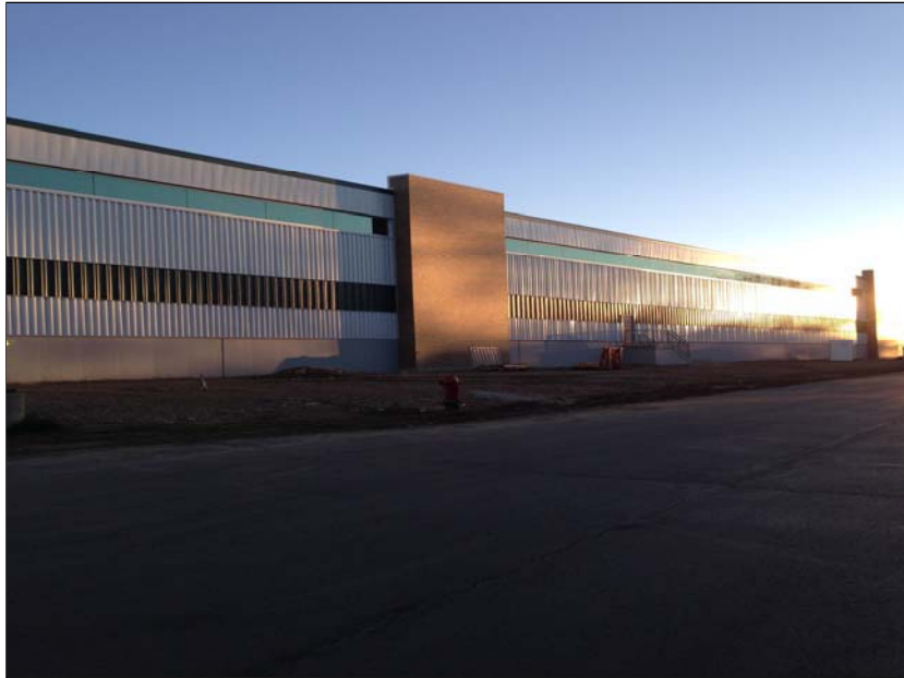
Photo 1: South side of building addition, looking east
