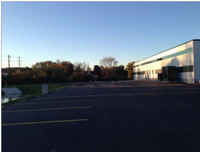
Photo 4: East side of building addition and paved parking areas, looking south
