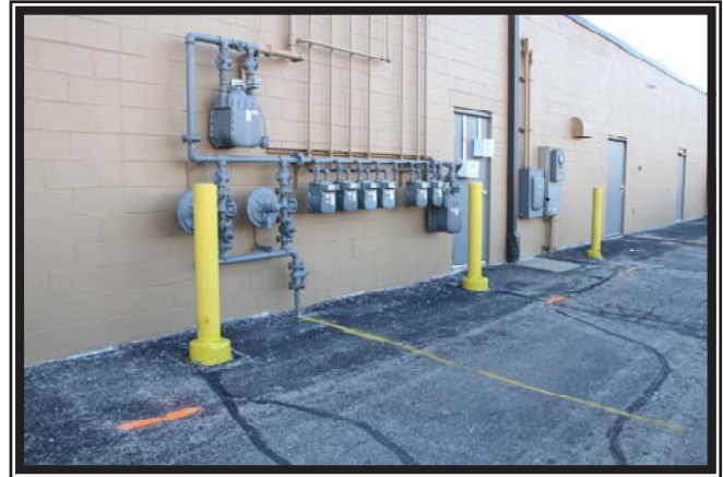
Photo 4 View of asphalt coving drive to rear of the Rainbow Cleaners and Planned Parenthood units.
