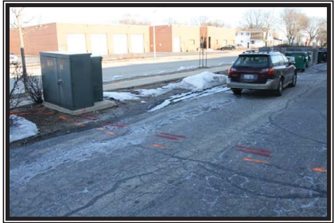
Photo 6 View of asphalt coving to rear of the Rainbow Cleaners, Relaxation Center, and Informed Choice units.
